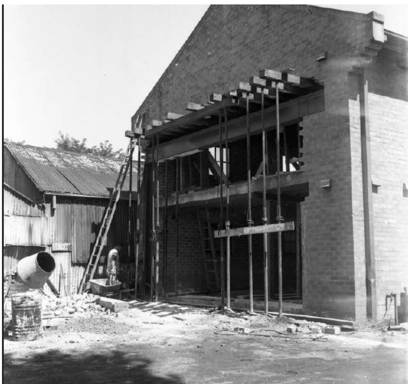
Figure 46 c1960s - New printing press in preparation at the Maitland Mercury office source: (D'Ombrain, n.d, fig 46).
