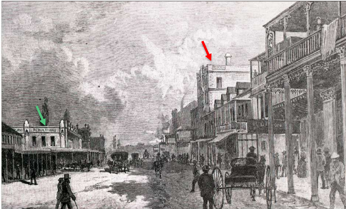
Figure 22 High Street, West Maitland, looking SE, [n.d] Newcastle City Library Bairstow, Damaris John Turner Collection source: (Bairstow, n.d. fig 22).
