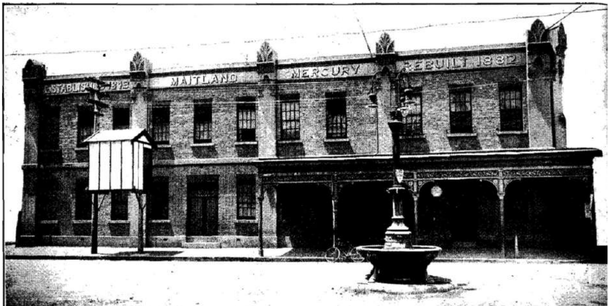
Figure 34 Souvenir book Back to Maitland Week, 7th to 12th November 1927 – pg22 The "Mercury" Buildings, West Maitland source: (Brock, 1927, p.22, fig 34).
