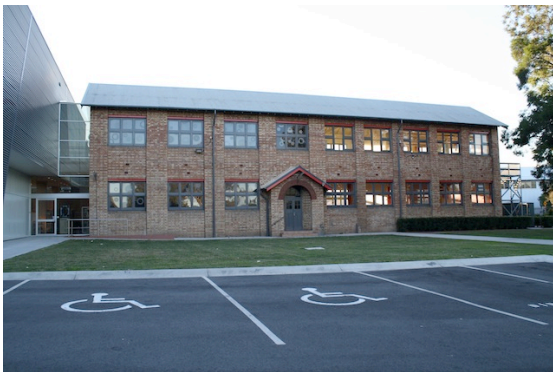
The Rear Building viewed from the adjacent vacant site on the south-east.
