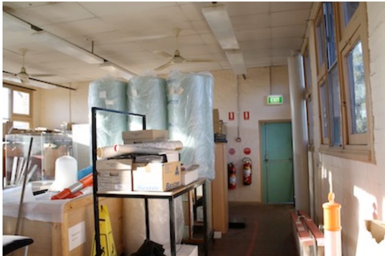
View of north east wall with fire escape door in background.
