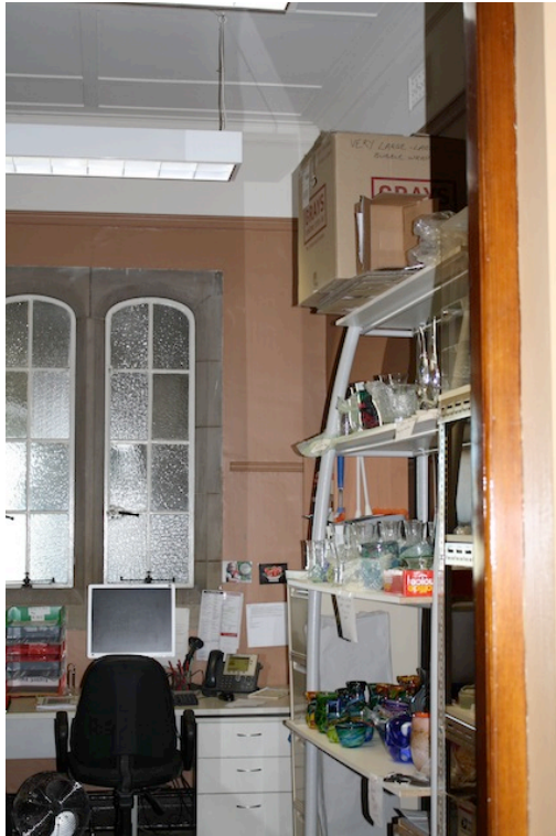
View of south west wall showing steel framed window set in sandstone reveal.
