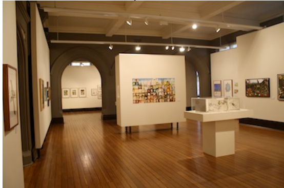
Rooms 6 &7 showing adaptation for new gallery use with partitions and opening of infilled pointed arches. Coffered ceiling is evident in photo.
