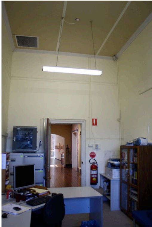
View toward north east wall with original ceiling concealed behind plasterboard
