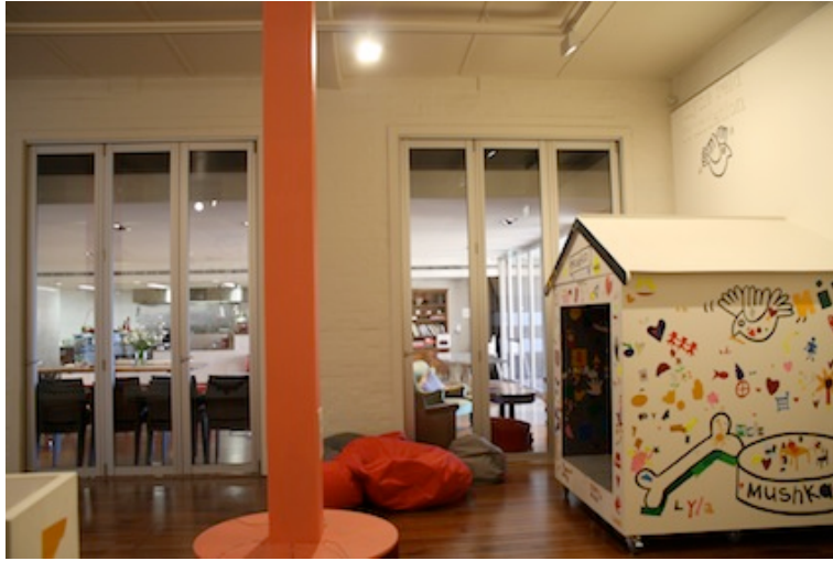
View toward north west wall with new aluminium concertina doors.
