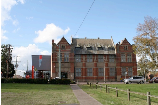
View of the High Street façade of the main building from the carpark and the vacant site directly opposite the MRAG to the south-west
