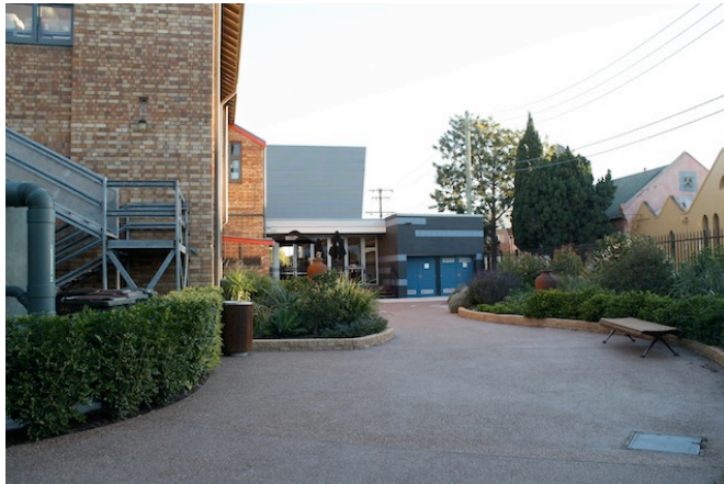
View of new landscape including new paving and planting on northern corner area of site.
