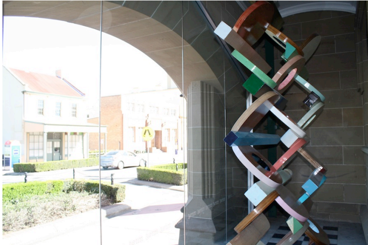
View toward south-west Corner showing new glazing to opening and artists installation
