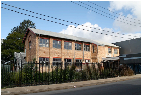
View of the Rear Building from James Street.
