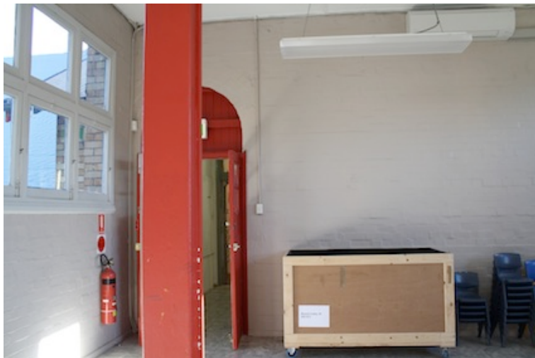
View toward south west wall with door to Entrance Hall. This wall differs from others in the bond pattern which is colonial bond. The door in this walls also differs from the flat arch doors in the rest of the building.
