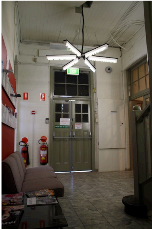
View toward south east wall showing original entrance door (now used as fire exit).
