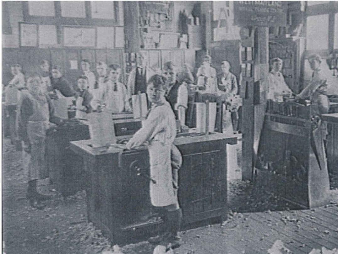
Figure 11 Interior Rear Building
