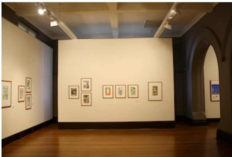
View toward south-west wall with new partition concealing perimeter wall behind
