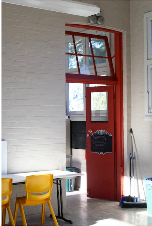
View of east corner with door to former Electricity Room.
