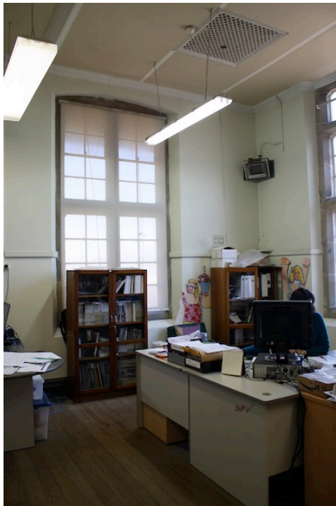
View of south corner with original ceiling concealed behind plasterboard.
