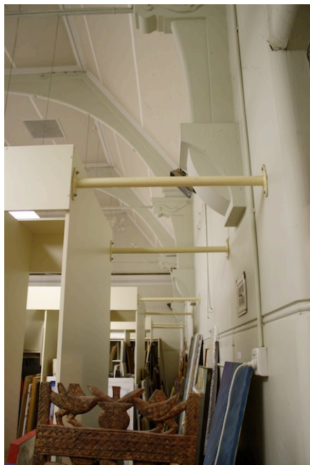
View along north-east wall showing anchoring of new storage units
