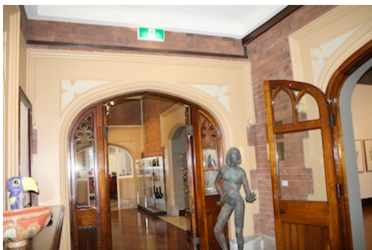
View of doors on north-east wall with the main staircase hall beyond
