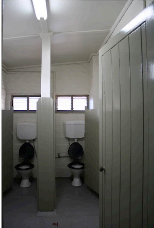
View toward north east wall of extension.
