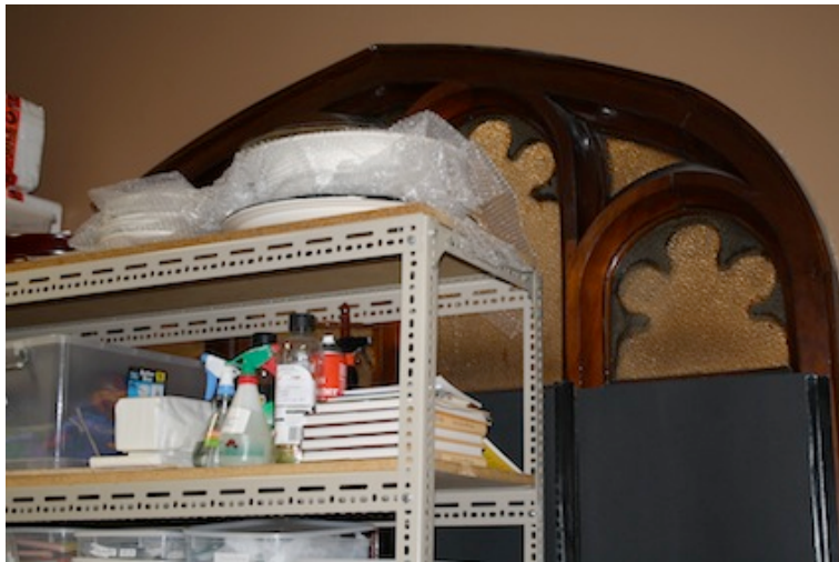
View south east wall showing the (now concealed) former counter window.
