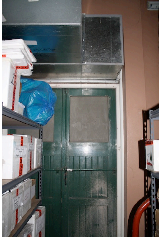
View of north-east wall showing new air conditioning ducting
