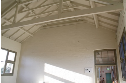
Room 24 showing the exposed queen post truss.
