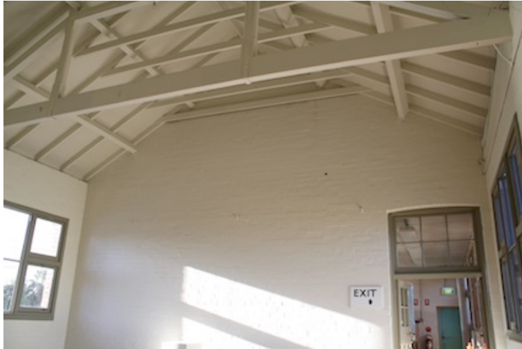
View of north east wall with door to former Plumbing Room
