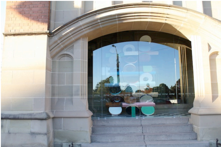
Original High Street Entry showing new fixed glazing
