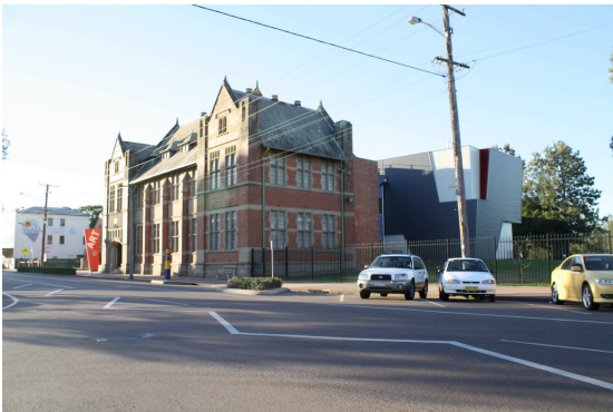
View of the Main Building from the south-east in High Street.
