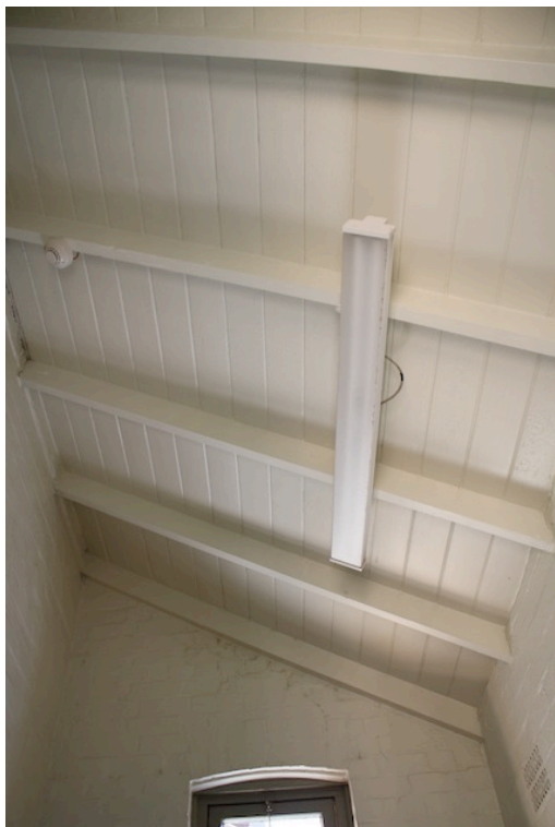
View of ceiling junction with south-west wall
