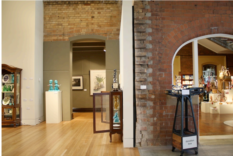
View of N end of facade with openings to corridor (left) and stair hall (right)
