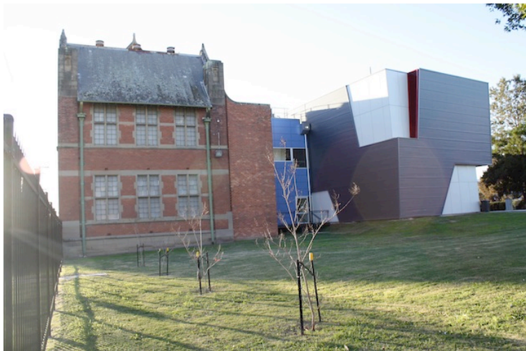
South-east elevation showing fire escape addition and the New Building (MRAG 2009)
