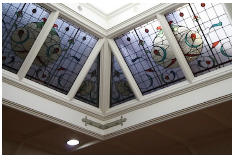
View of north corner of Art Nouveau lantern glazing
