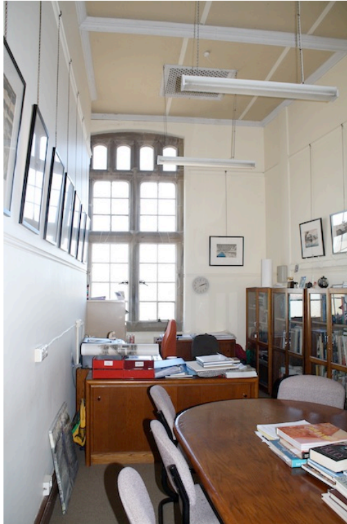
View toward south west wall with original ceiling concealed behind plasterboard
