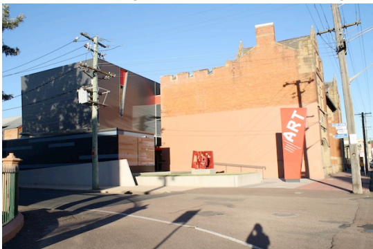
View of north-west elevation showing new MRAG building and glazed connection.
