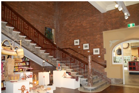
Staircase showing the use of contrasting materials and the simple detailing of the newel post.
