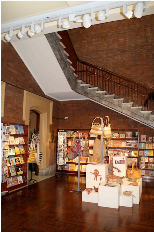
View of west corner of Stair Hall showing cantilevered marble staircase
