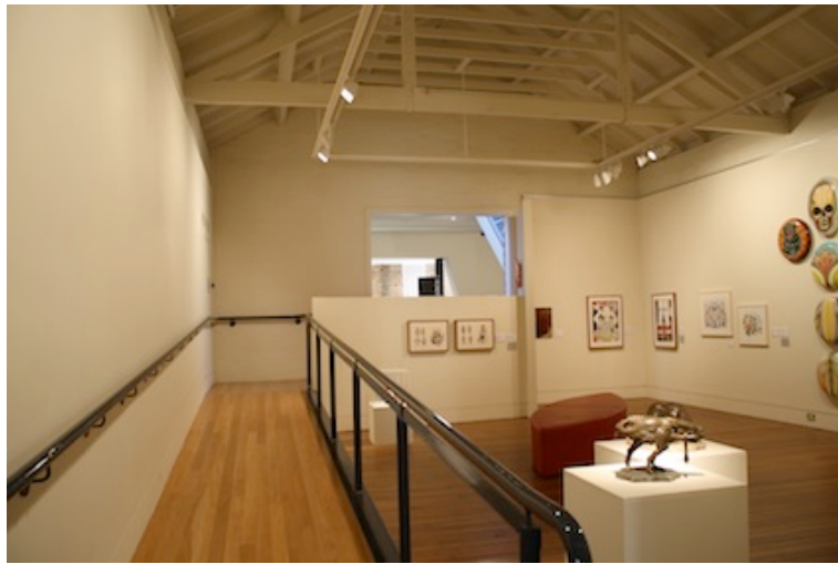
View toward south west wall showing new opening and new ramp.
