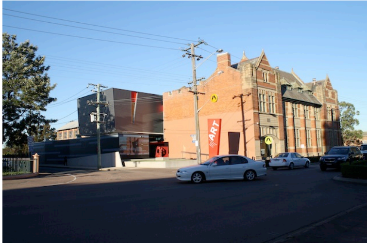
North-west elevation with the Rear Building just visible (to the left of the new building)
