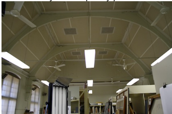
View showing hammerbeam trusses and temporary plasterboard ceiling in room13.
