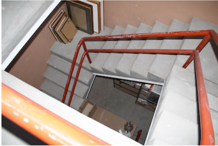
View toward south east wall of ground floor.
