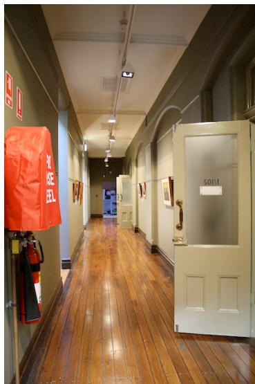
View toward south east wall showing new track lighting
