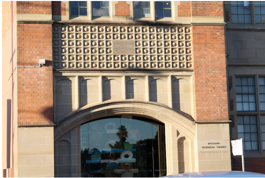
Original entrance with a segmental arch, carved mouldings and simply decorated spandrel.
