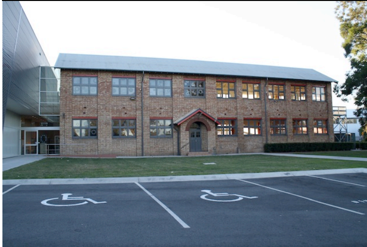
South-east elevation of Rear Building and the new connection to the Gallery building.
