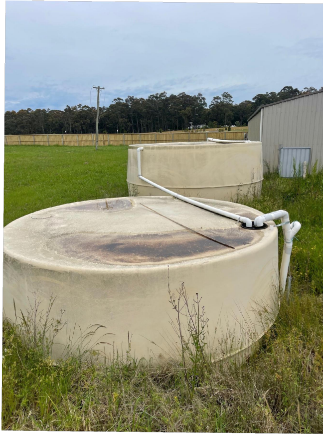
Photo 5: View of the water tanks in the centre of the Site. Taken on 7/10/2020.
