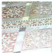
FT Existing Floor Tiles
