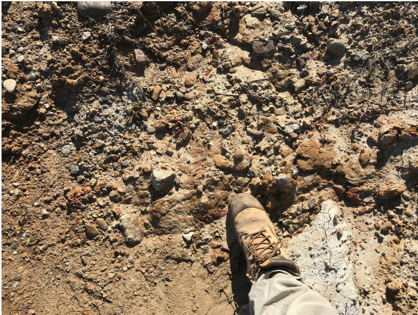
Photograph 3 – Example of outcropping bedrock on the batter slope in the northern portion of the site
