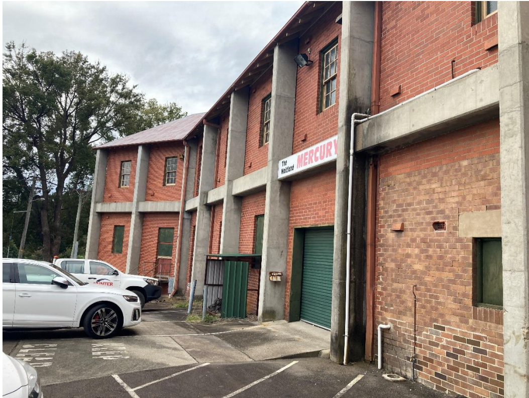
Photograph 5 – Rear of building adjacent carpark
