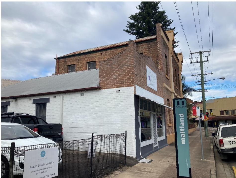
Photograph 2 – Western facing commercial front
