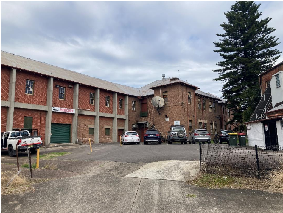
Photograph 1 – Site rear carpark and rear of building
