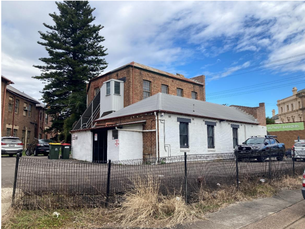
Photograph 3 – Rear of western facing commercial front
