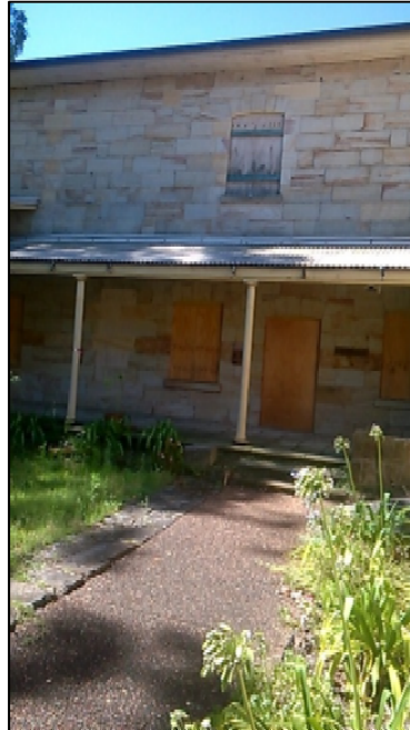
Figure 3: Sandstone block construction
