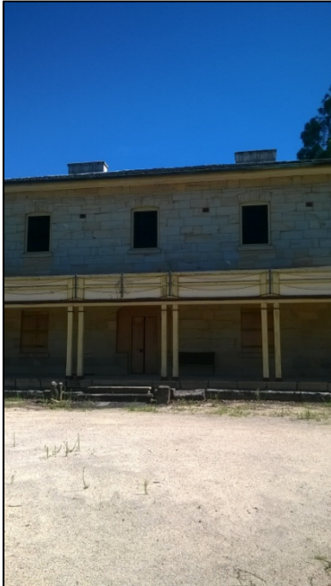
Figure 2: Side view of Closebourne House
