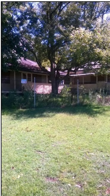
Figure 4: Existing timber buildings
