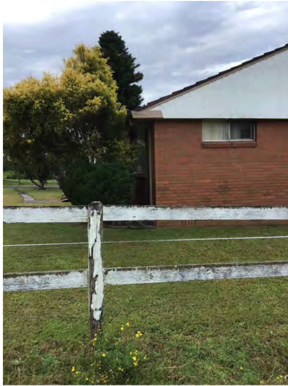
Photo 7: View of existing residential structure (facing north-east)
