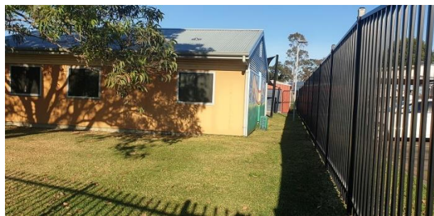
Photograph 6 From northeast of “D Block”, beside eastern boundary, facing west.
