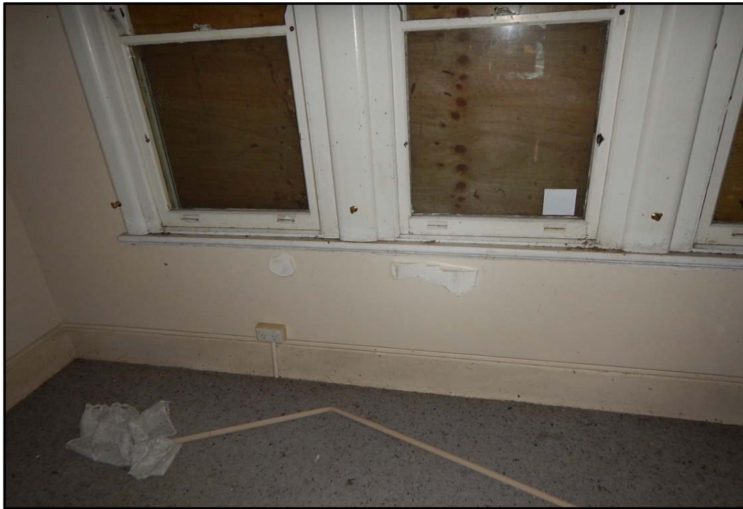
Photo 23: Building 13 - Interior beige paint
