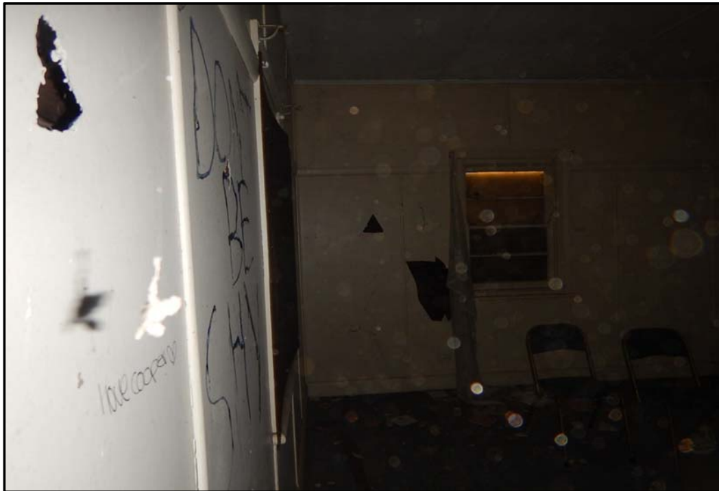
Photo 5: Building 11 - Wall sheeting in Bed 1
