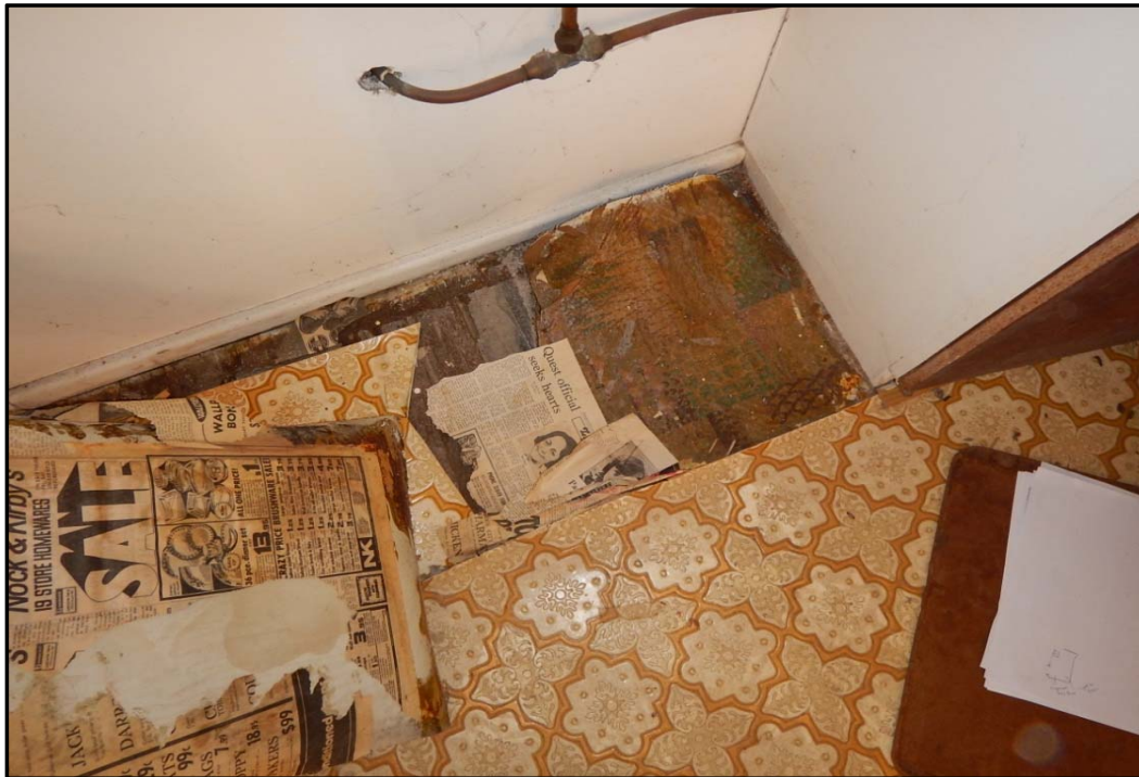
Photo 19: Building 13 - Vinyl flooring in lower Room 1
