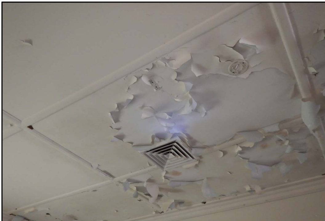
Photo 26: Building 13 - Beige paint on ceiling in upper floor landing
