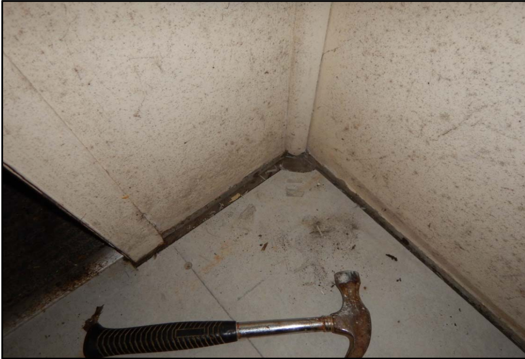
Photo 7: Building 11 - Toilet wall sheets
