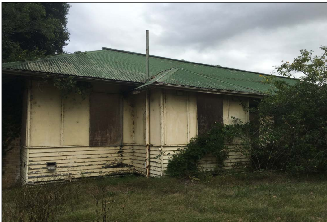
Photo 29: Building 14 - External building cladding comprising ACM, looking south
