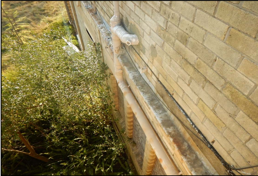
Photo 27: Building 13 - Lead flashing and damp course
