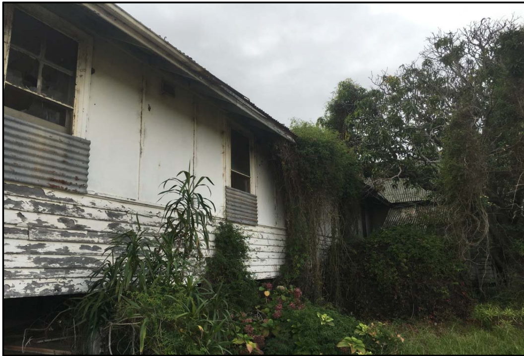
Photo 28: Building 14 - External building cladding comprising ACM, looking north east
