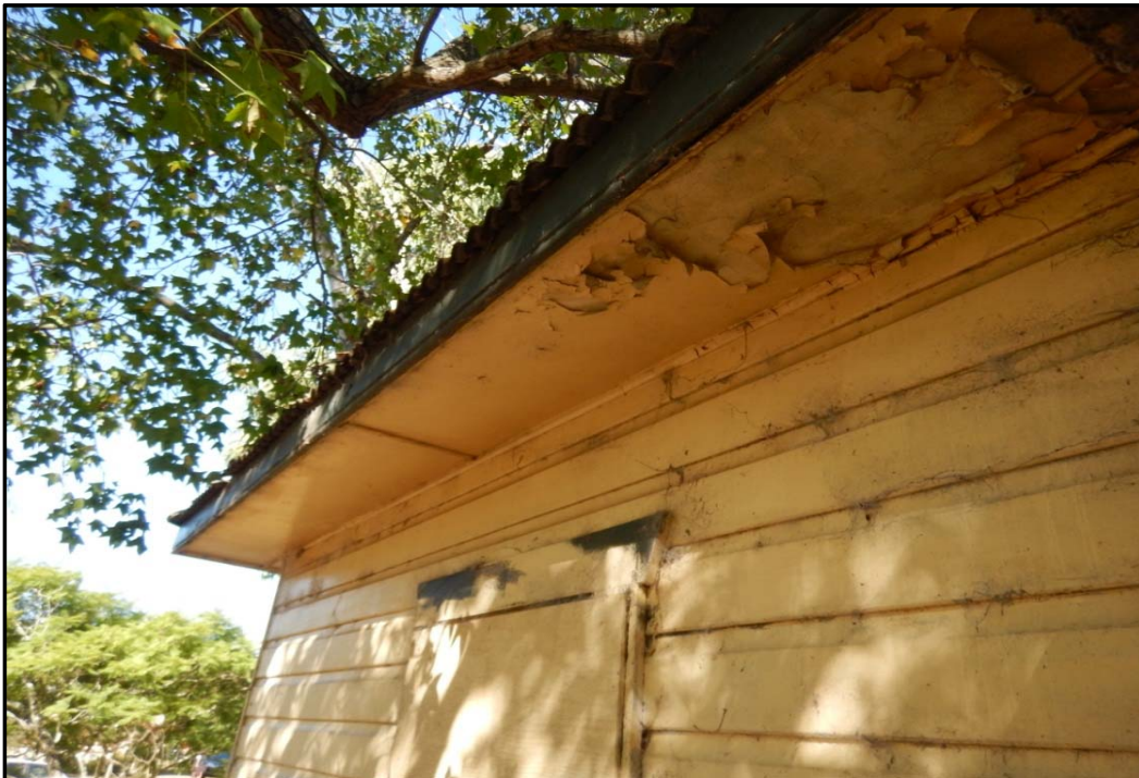
Photo 8: Building 11 - External Eaves
