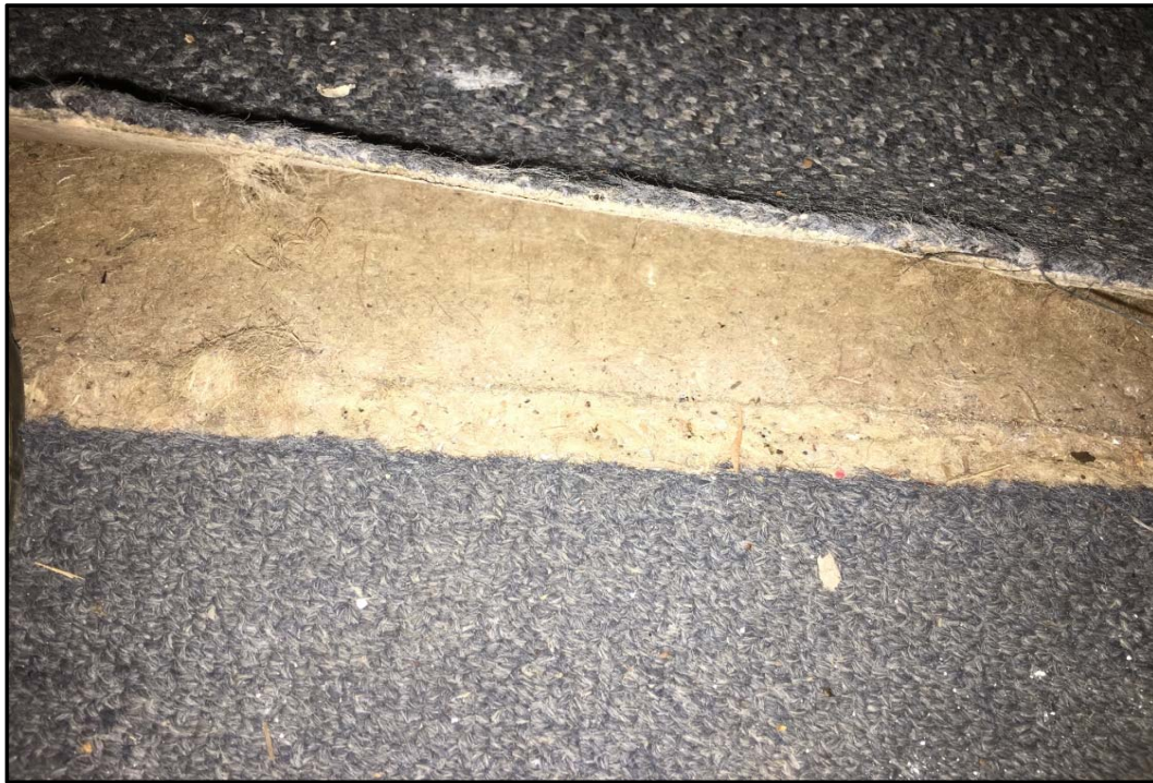
Photo 16: Brown SMF underlay under carpeted areas
