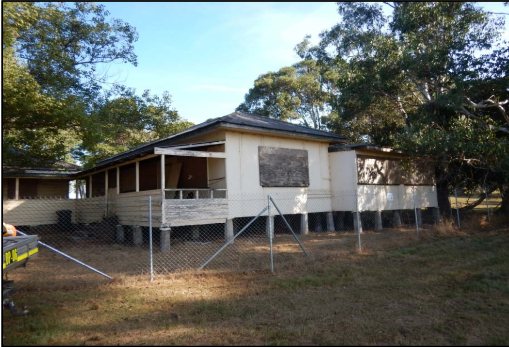
Photo 3: Buildings 10 and 11 - Asbestos corrugated roofing
