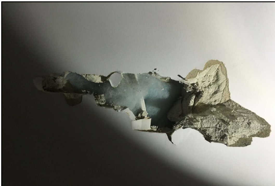
Photo 17: Insulation filling between internal wall cavities
