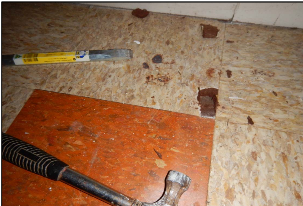
Photo 6: Building 11 - Vinyl flooring sheets in kitchen
