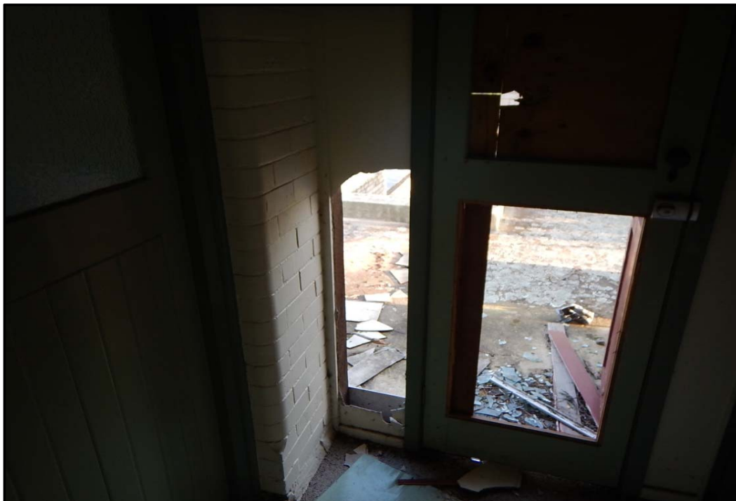
Photo 20: Building 13 - Exterior wall in access to livable roof space
