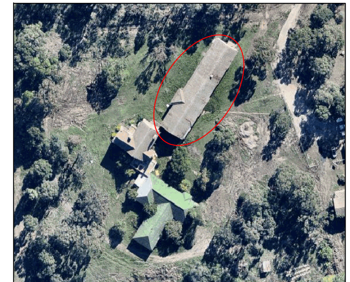
Aerial View of Site
