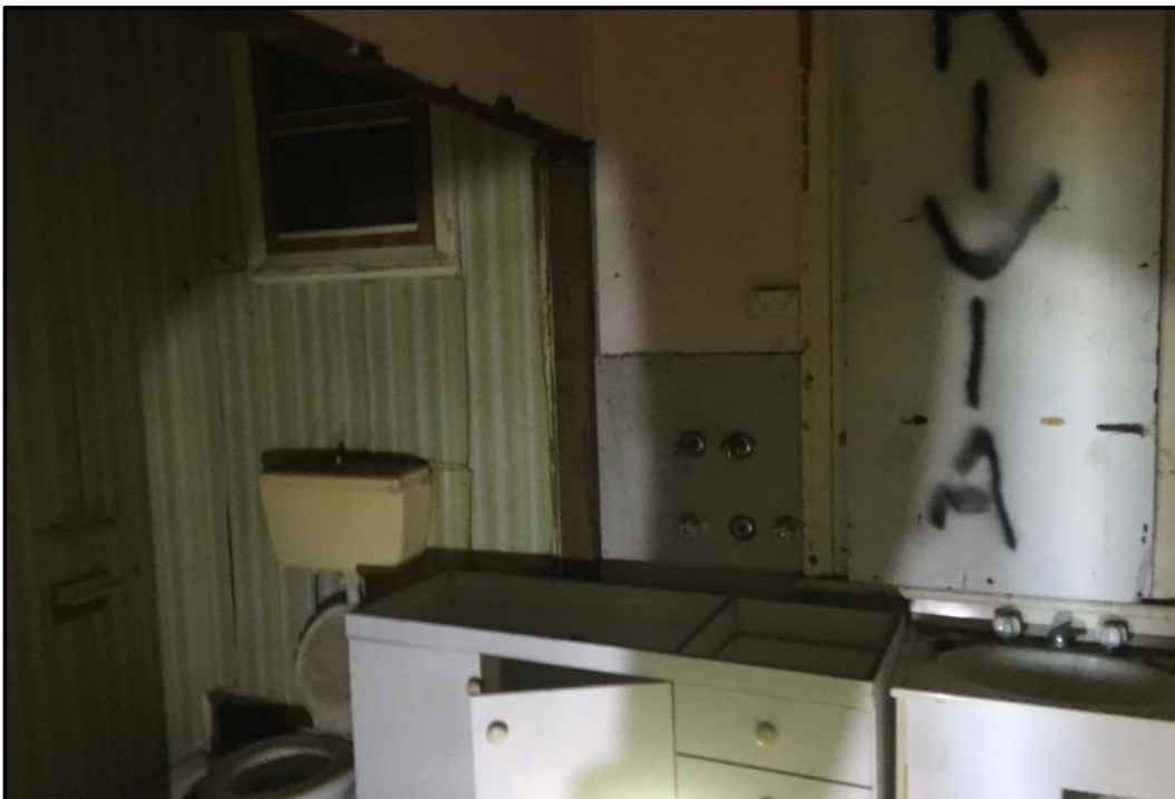
Photo 31: Building 14 - Internal wall linings, comprising ACM in bathroom area
