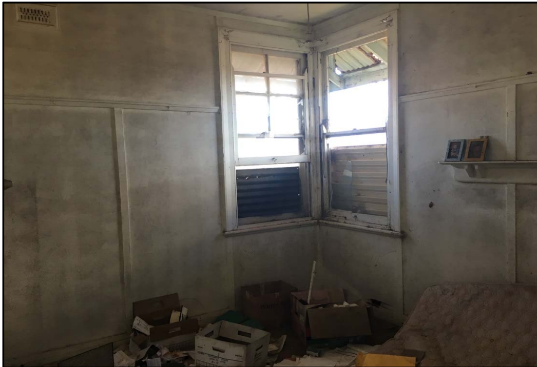
Photo 32: Building 14 - Internal wall lining, comprising ACM in rooms
