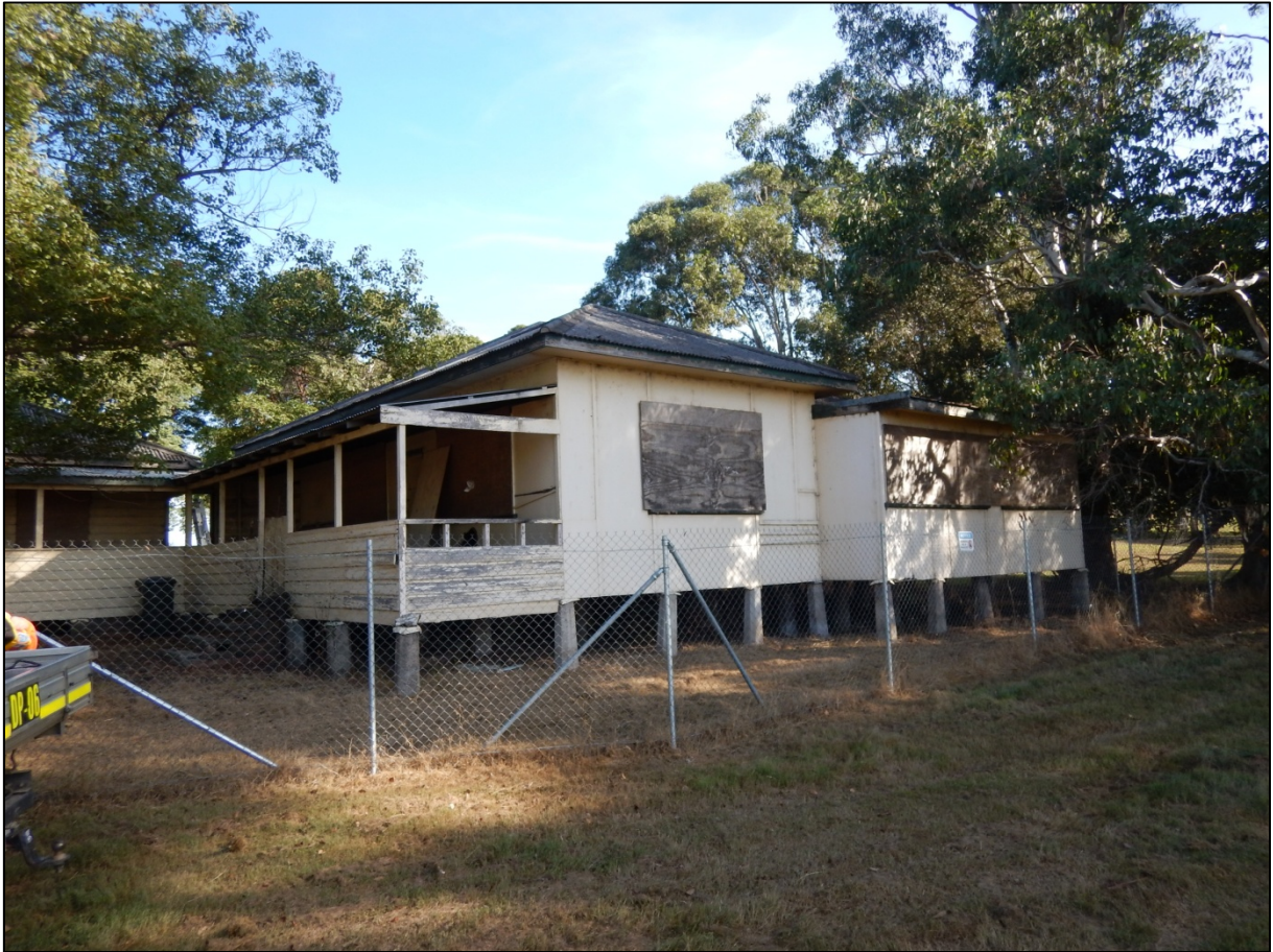
Figure 3: View of Buildings 10 and 11
