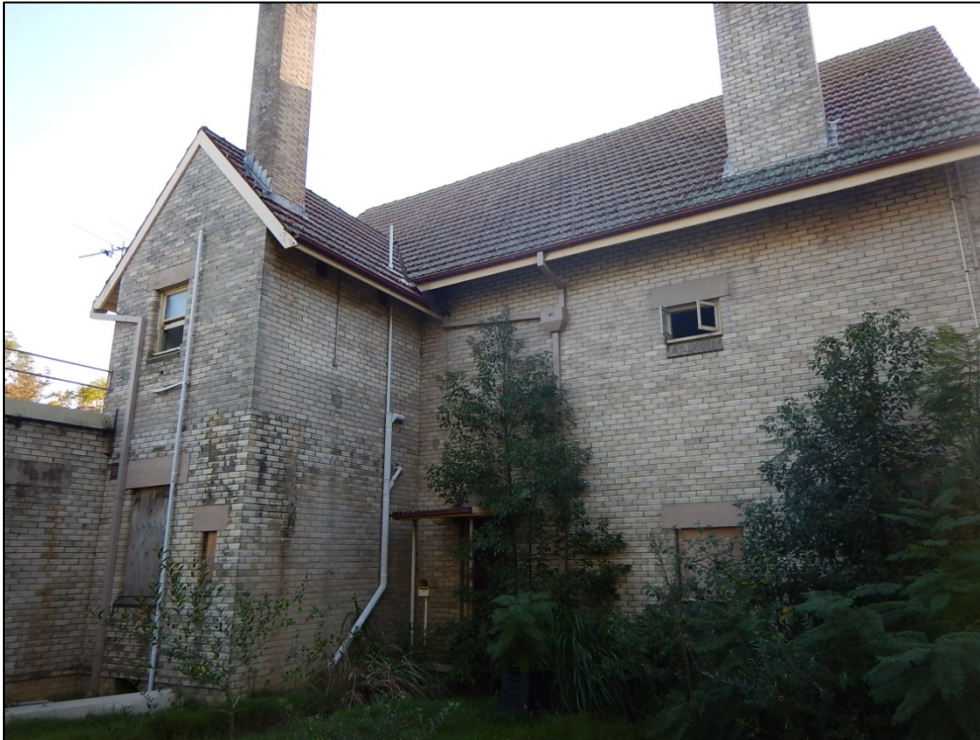
Figure 5: Eastern frontage of Building 13
