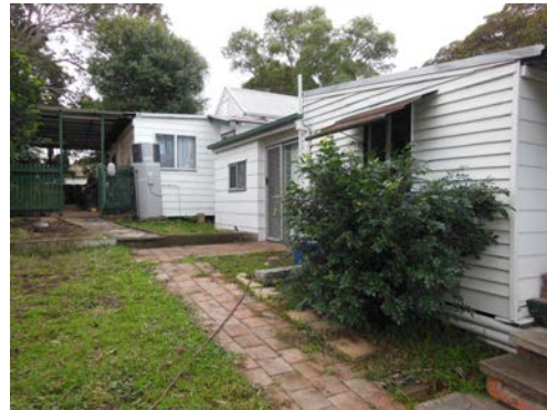
Figure 22: South elevation showing the successive and disparate additions. Source: Paul Ackroyd
