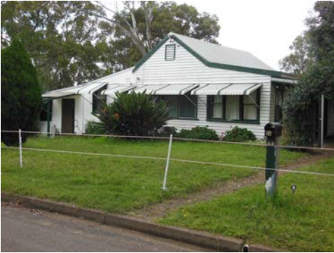
Figure 20: North eastern view of the cottage #54. Source: Paul Ackroyd
