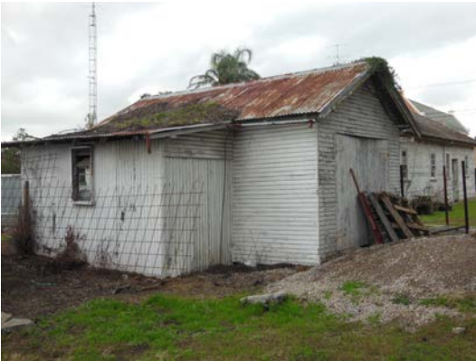
Figure 17: South east elevation of Garage. Source: Paul Ackroyd
