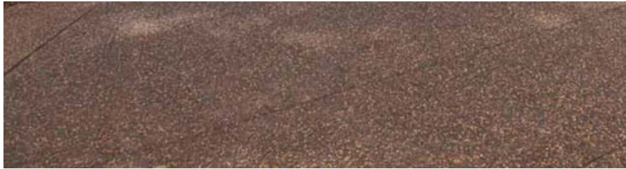
Figure 31. Concrete finish equivalent to "Morpeth Mix".
