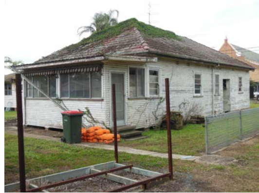
Figure 16: South east elevation. Source: Paul Ackroyd
