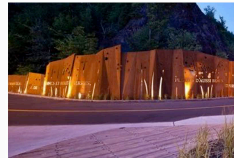
Corten facade treatment
