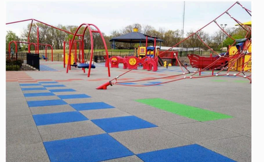
Rubber tile beneath play structure
