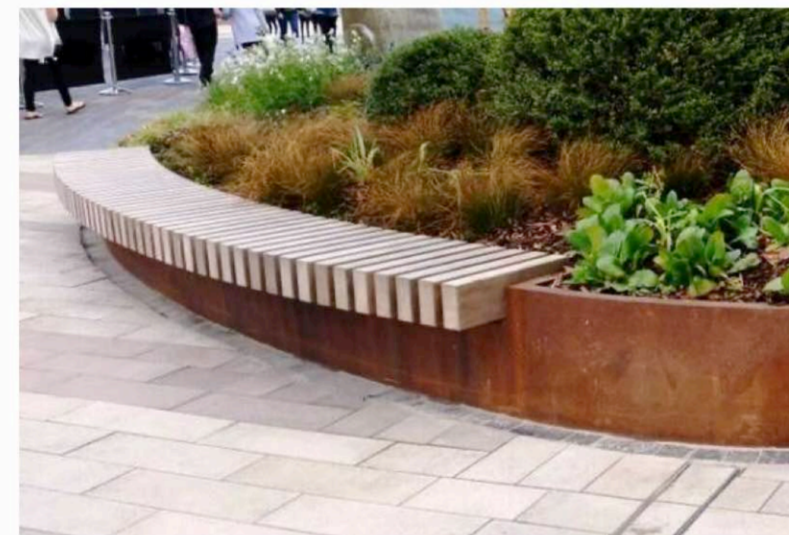
Corten retaining with mounded planting and floating timber seat
