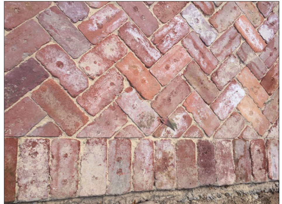
Recycled brick pavement to pathways & courtyard - Header course edge with 45 degree herringbone pattern
