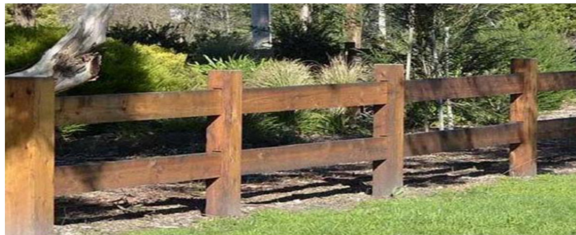
Timber post and rail boundary fence
