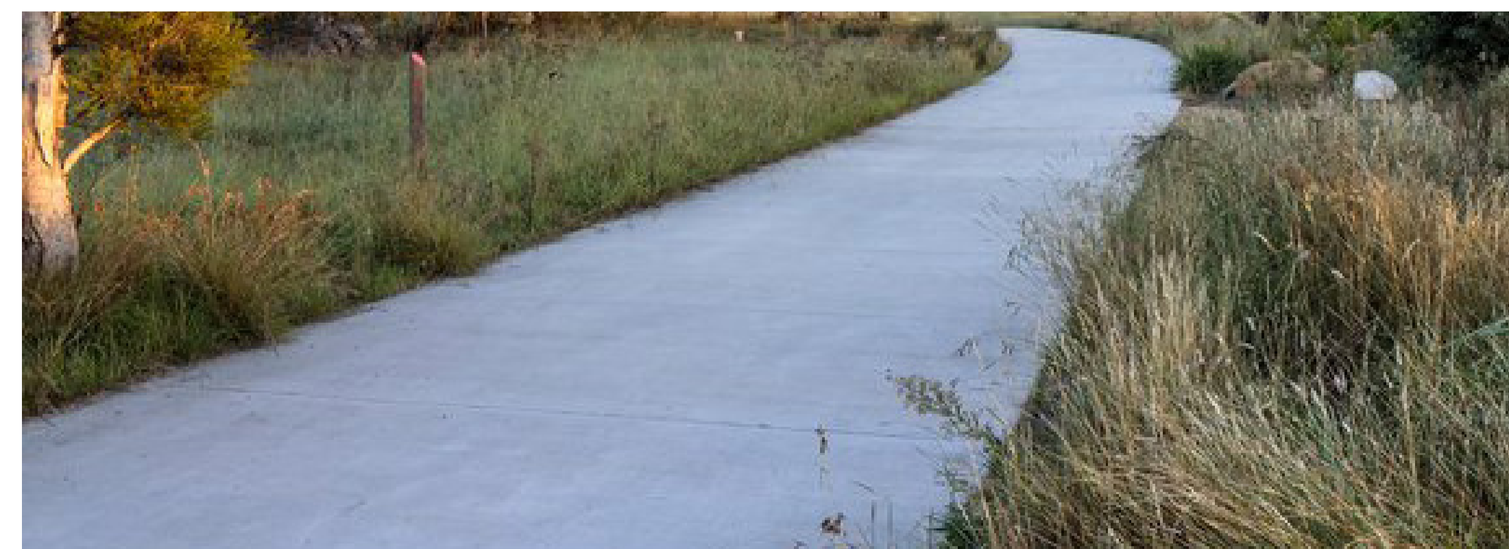
Concrete Pedestrian Footpath
