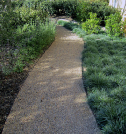
Decomposed granite footpath
