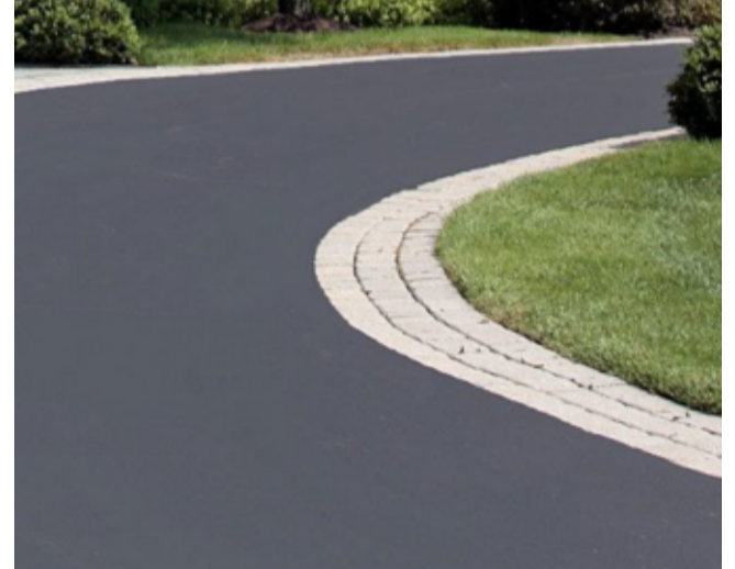
Hot mix asphalt pavement
