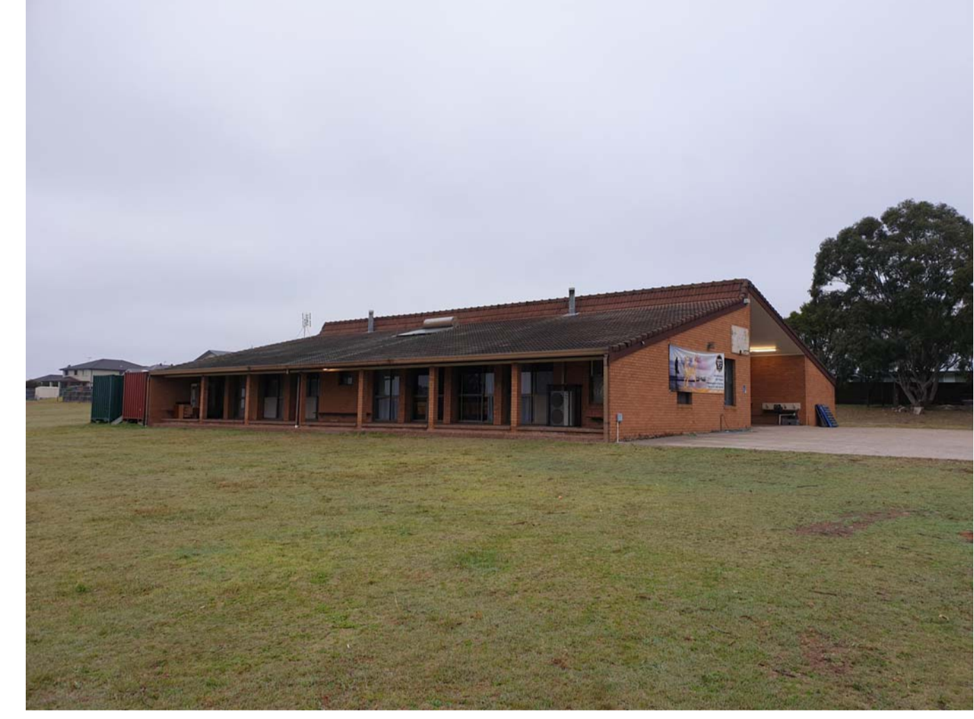
PHOTO 05: View of existing classroom building
