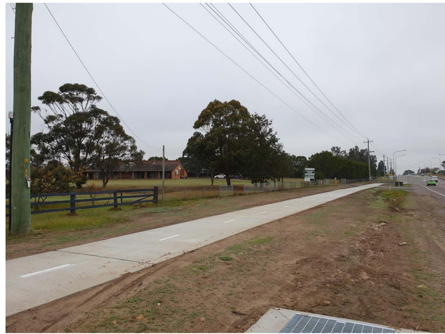
PHOTO 01: View of school from Cessnock Road
