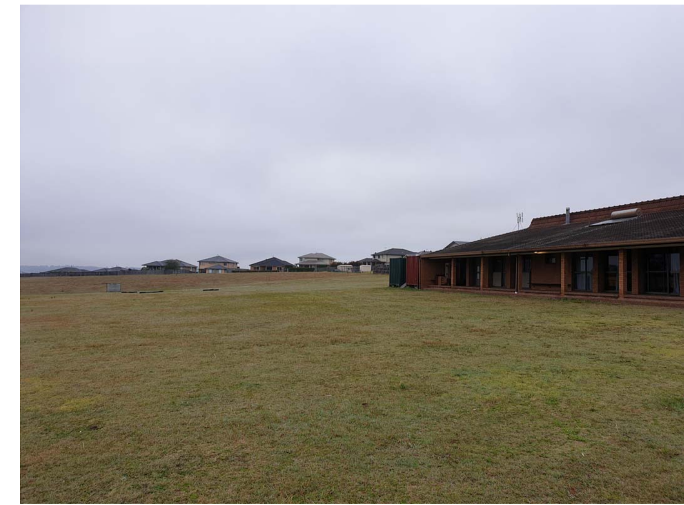
PHOTO 06: View of existing classroom building and location of proposed work
