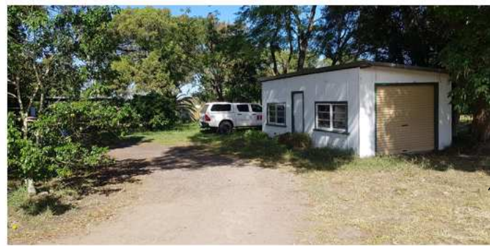
EXISTING STRUCTURES ON 54 BONAR STREET
