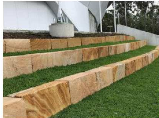
SANDSTONE BLOCK RETAINING WALL
