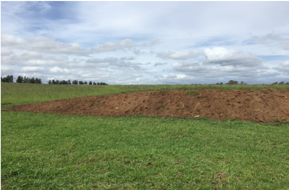
Photograph 2: Stockpile of soil on Lot 32
