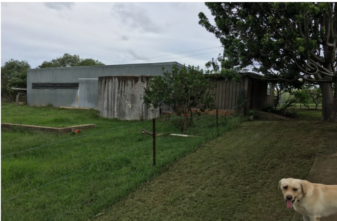
Photograph 4: Shed and water tank on Lot 2
