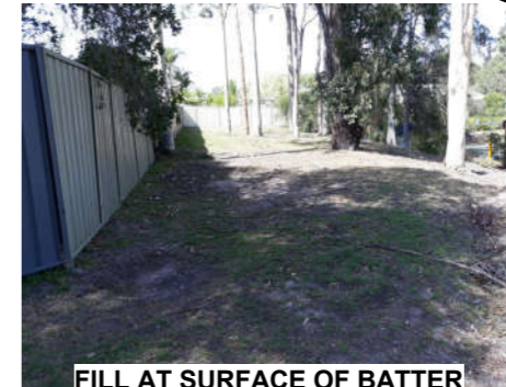
FILL AT SURFACE OF BATTER
