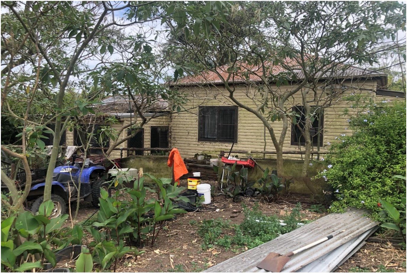
Photograph 1 - Residential dwelling - northern portion of the site
