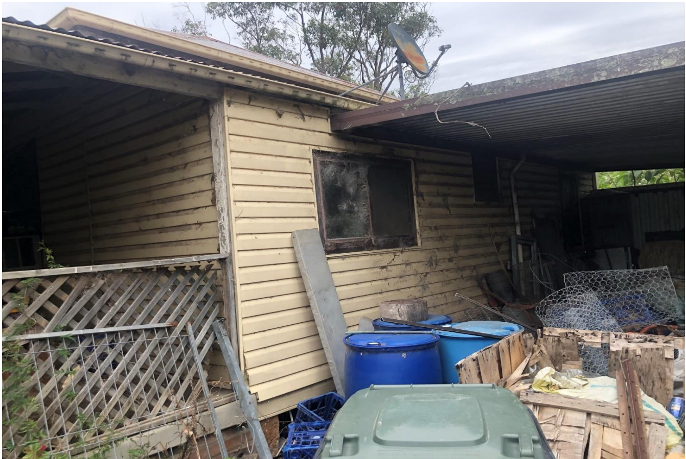
Photograph 2 - Showing carport - north of residential dwelling
