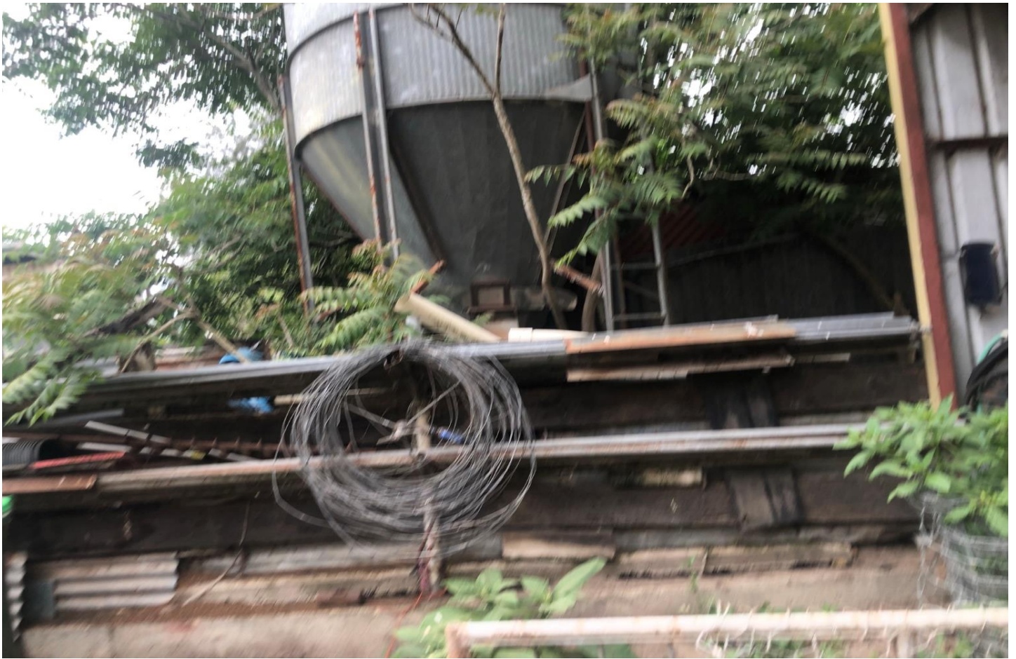
Photograph 19 - Metal grain silo
