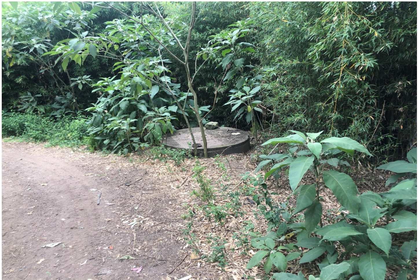
Photograph 5 - Showing septic tank and overgrown soakaway area
