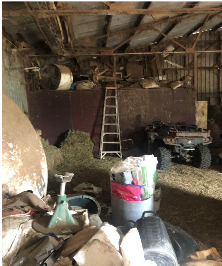
Photograph 8 - Shed 2 - hay bales, quad motorbike, plastic, metal etc
