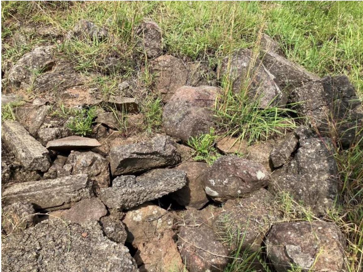
Photograph 9: Remnant building rubble from retaining wall demolition (Lot 1308).
