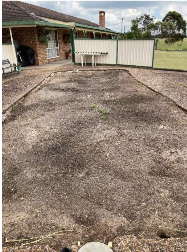
Photograph 3: Leisure pool filled with imported fill.
