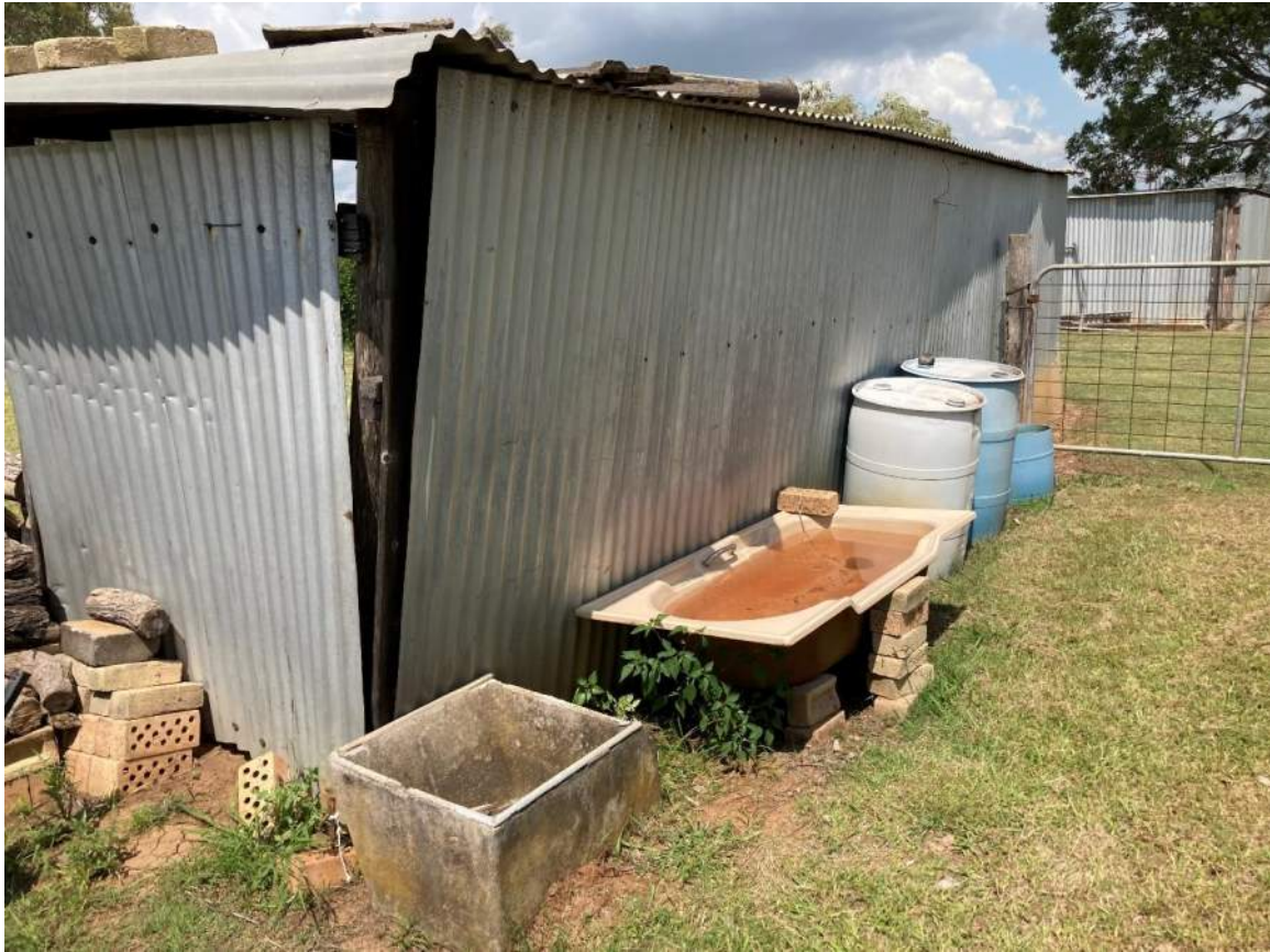
Photograph 7: Farm storage shed on Lot 1308.
