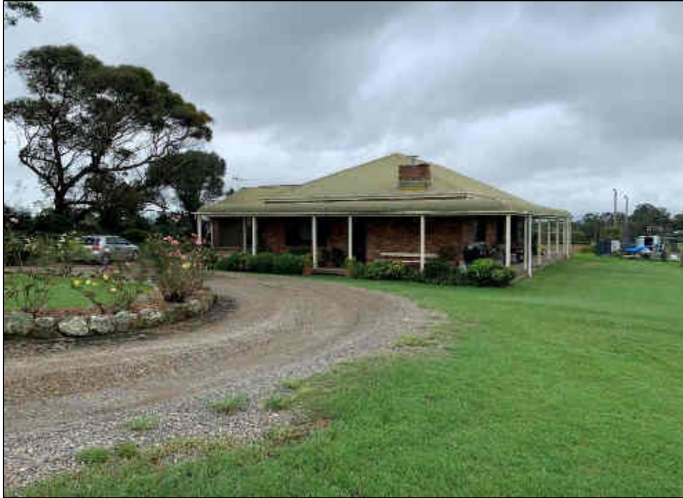
Photograph 1: The residential dwelling viewed from the southeast.
