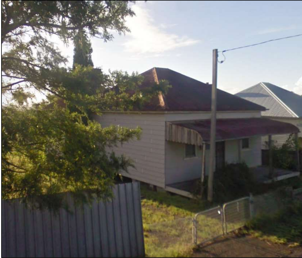
Photograph 1: 21 Owlpen Lane, Farley, NSW 2320, viewed from the northwest of the dwelling.
