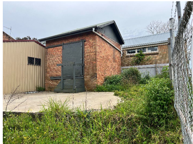
Eastern view of the back portion of 75 Elgin, highlighting external structure and visible from Napoleon Lane
