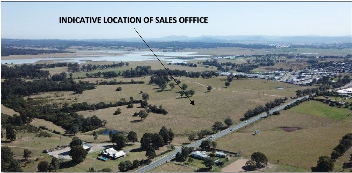
Plate 1: The proposed development will be constructed within Stage 1 of Precinct 1A
