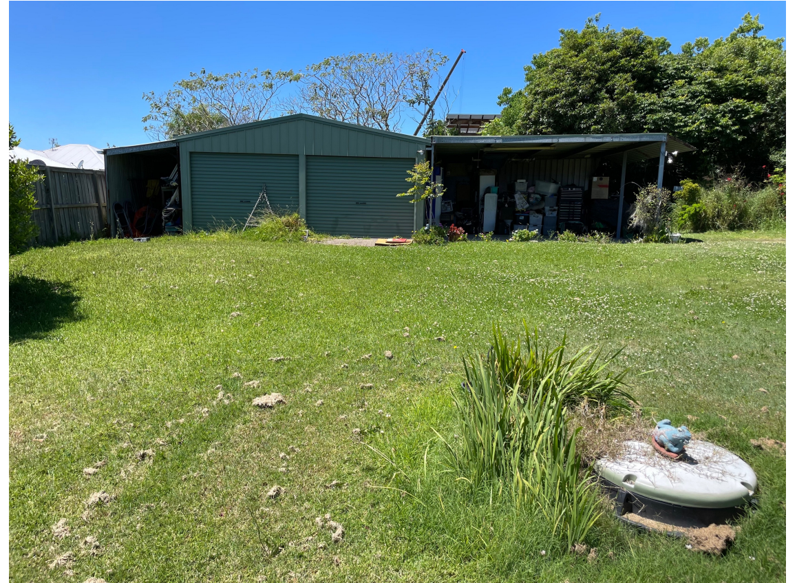
Figure 11. The septic tank and steel paneled shed.
