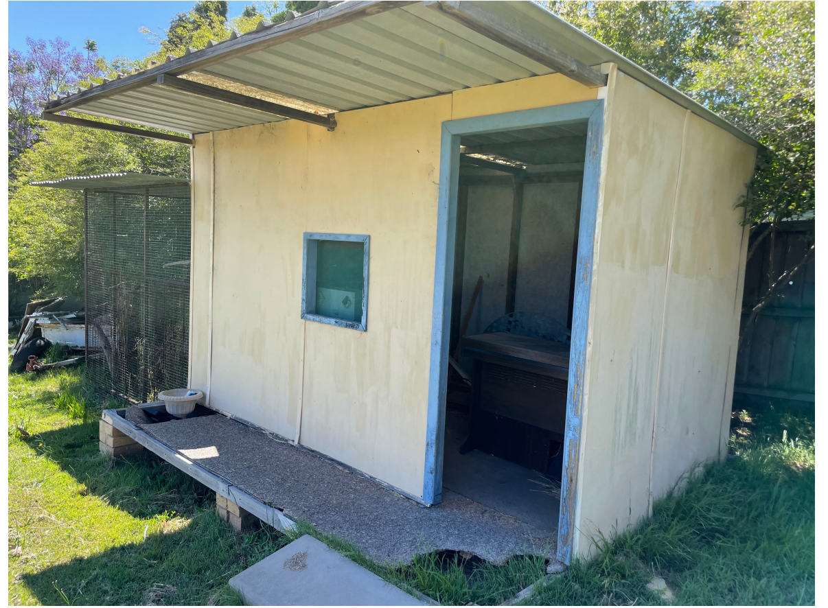
Figure 9. The fibro shed near the southern site border.
