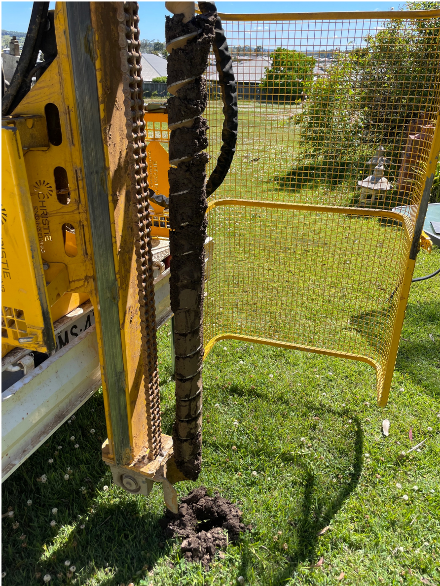
Figure 10. The site features a silty clay fill material, underlain by a dense moist clay.
