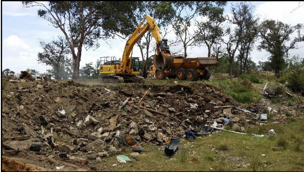
Print 11 Excavation start of South-Western Fill Zone.
