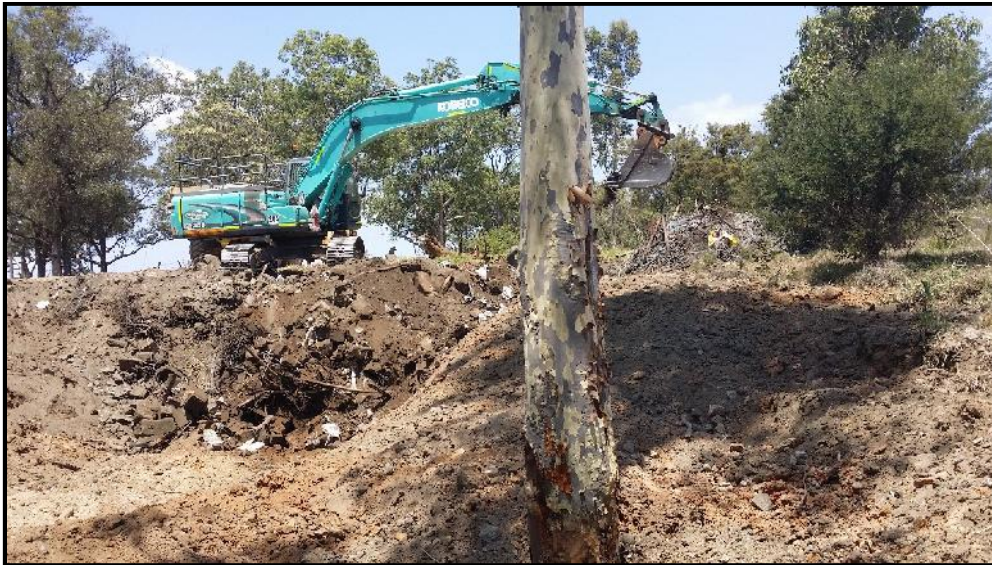
Print 6 Excavation of Western Fill Zone.
