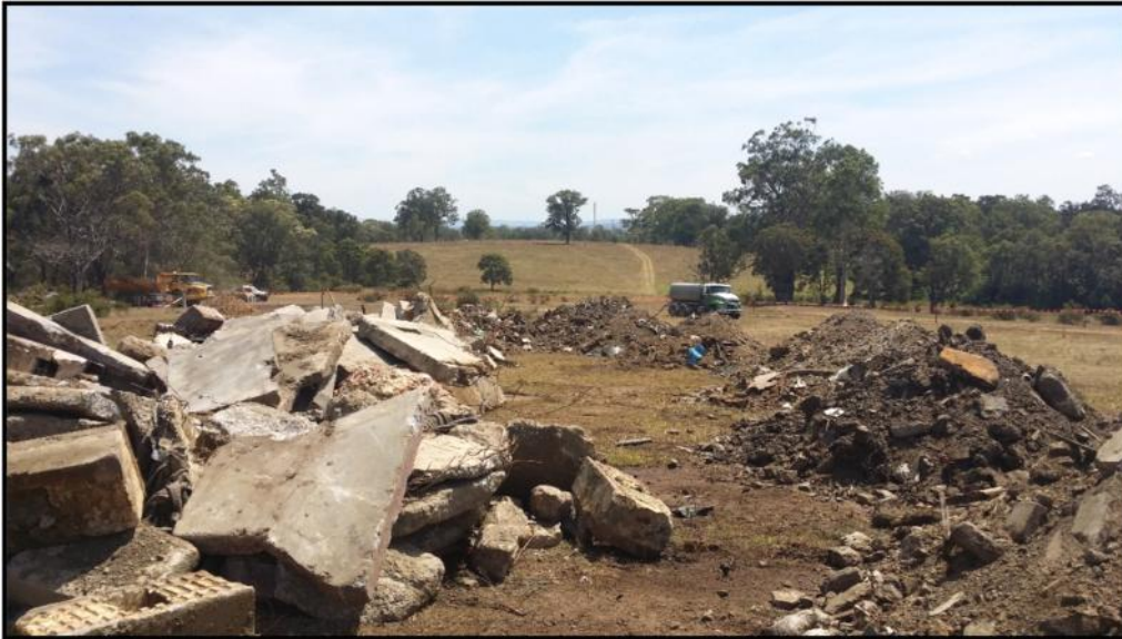
Print 5 Main Staging area with material from western fill zone.
