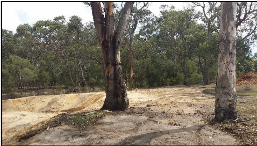
Print 6 Excavation of Western Fill Zone.
