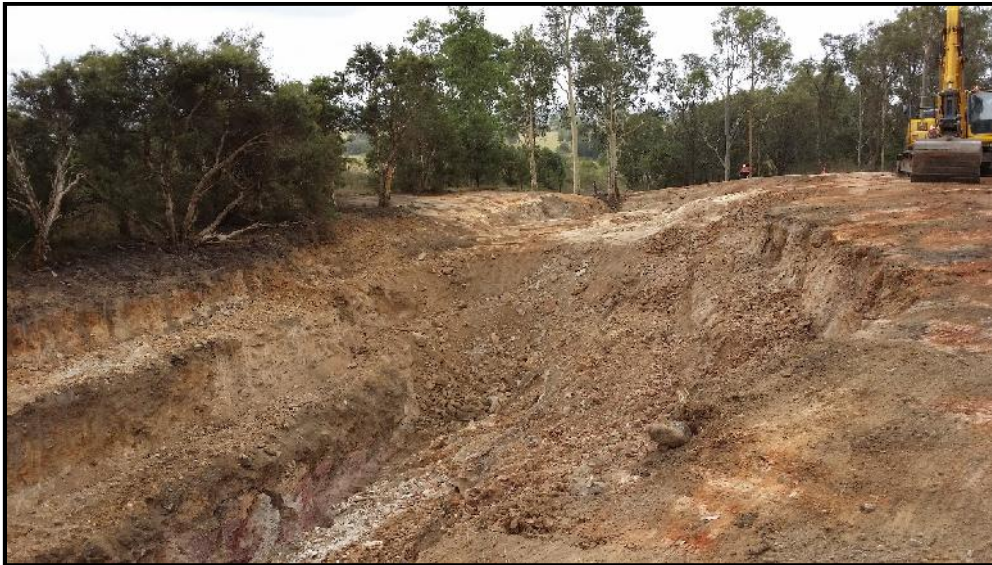
Print 10 Southern end of WFZ looking north following benching.
