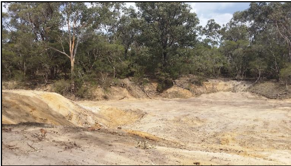
Print 6 Excavation of Western Fill Zone.
