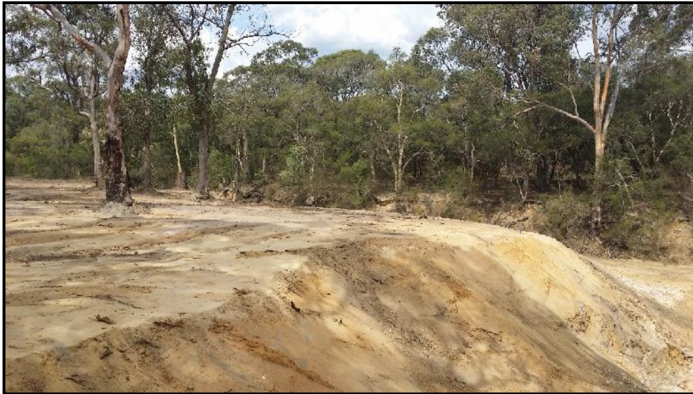
Print 8 Middle excavation section of Western Fill Zone.
