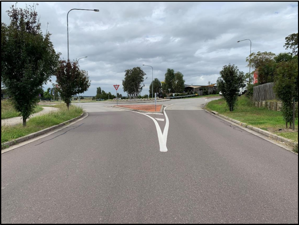
Photo 1 – Looking east along Thorncliffe Avenue towards intersection with Government Road
