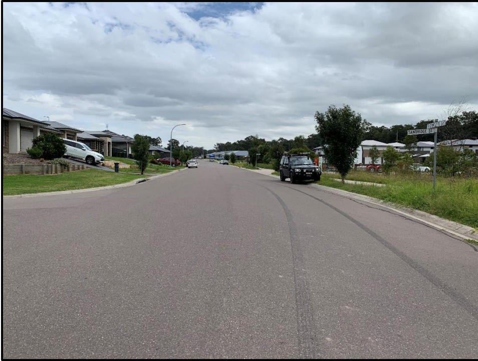
Photo 3 –View west along Thornclyffe Avenue showing typical cross section
