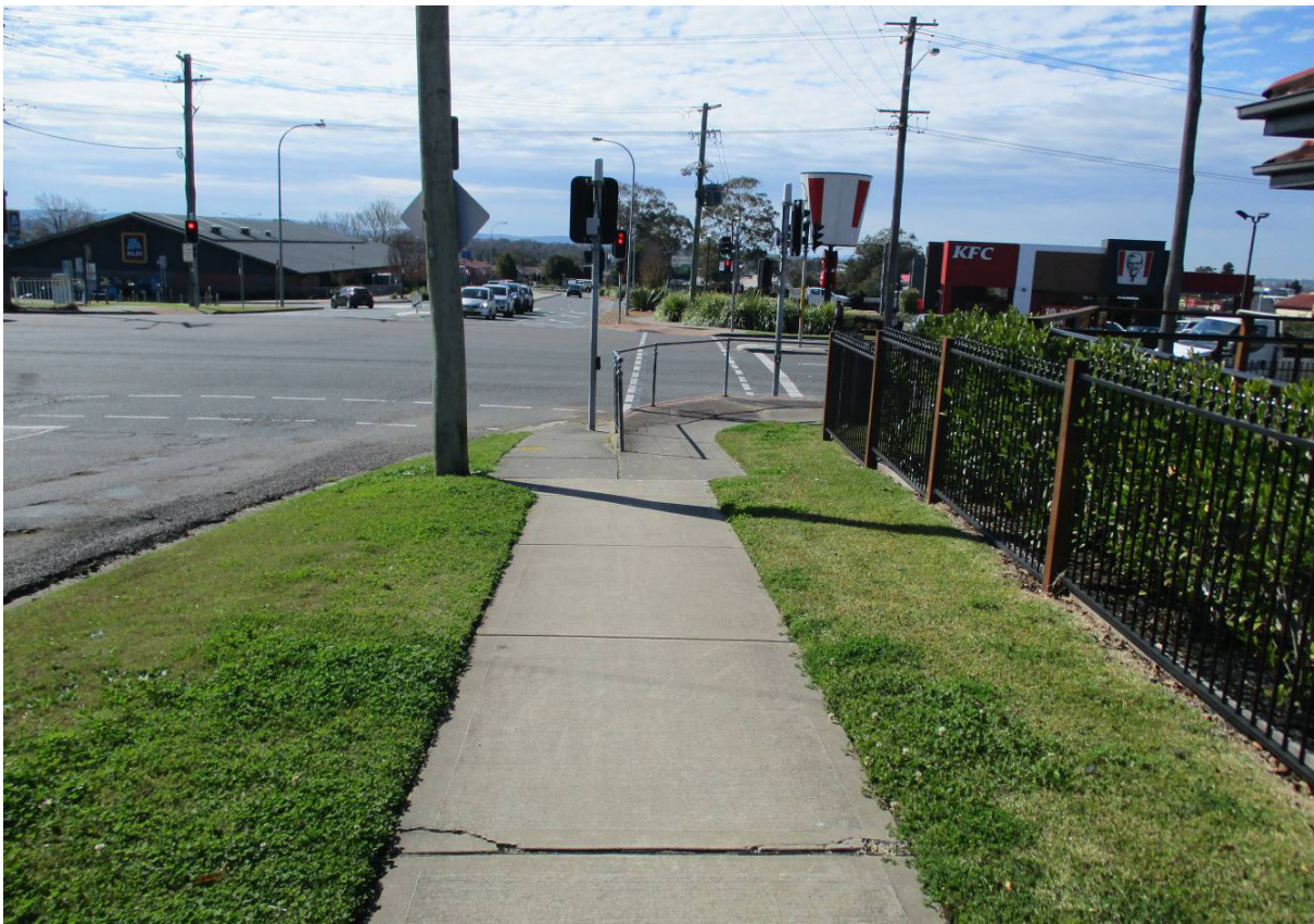
Photograph 7 – Pedestrian crossing phases New England Highway at Arthur Street
