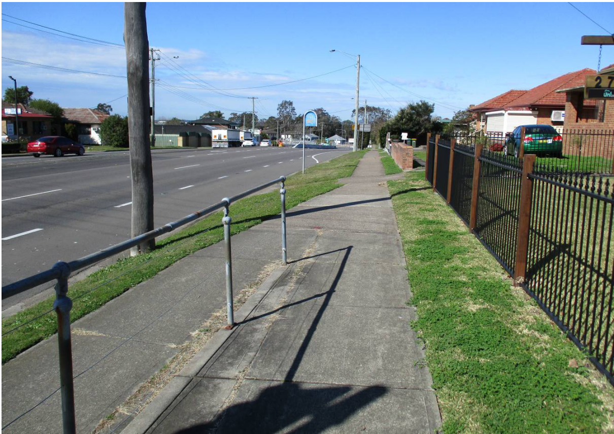
Photograph 6 – Bus Stop and Footpaths – New England Highway – site frontage
