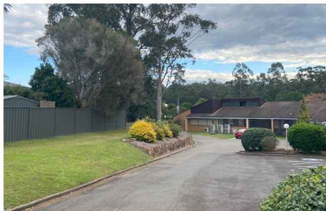
Figure 6 Existing RACF facility and back of house loading area
