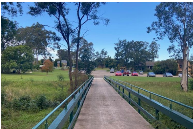
Figure 5 Existing at-grade car park as viewed from the pedestrian link bridge
