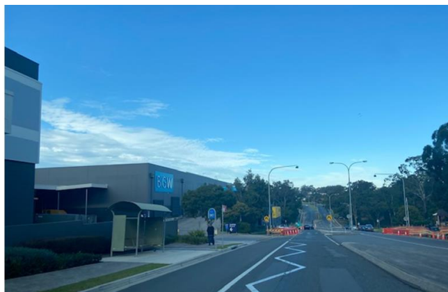
Figure 8 Green Hills Stockland Shopping Village as viewed from Stronach Avenue
