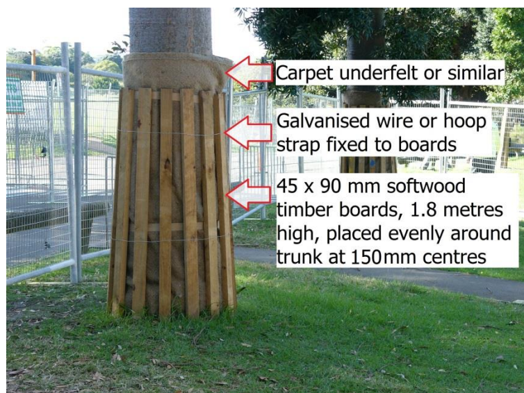
Figure 3 – Detail of Trunk Protection
