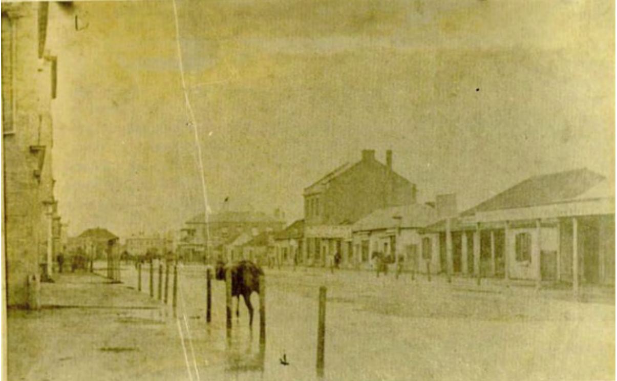
Figure 6: The Town Hall Café is the two storey building in the centre of the image of High Street West Maitland from 1868. Source National Library of Australia.
