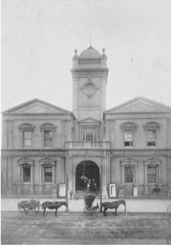
Figure 29: Maitland Town Hall. Source Newcastle Museum F A Cadell Collection.
