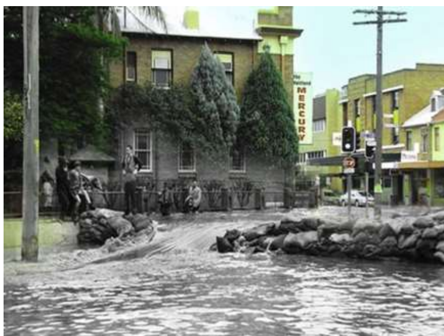
FIGURE 3.3 -1955 FLOOD AT MERCURY CORNER OVERLAYED WITH RECENT PHOTOGRAPH. PRESENT COUNCIL ADMINISTRATION BUILDING VISIBLE CENTRE RIGHT. Source: Flickr
