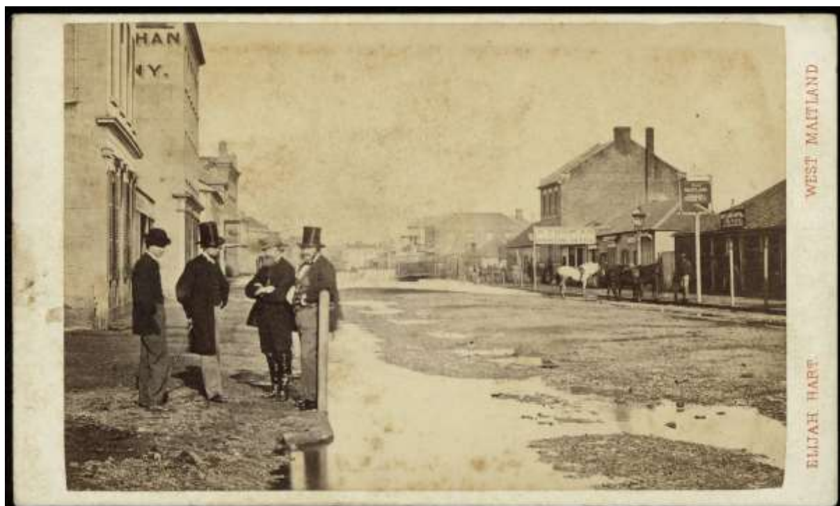
FIGURE 2.10 - HIGH STREET, WEST MAITLAND CIRCA 1870 FLOOD SHOWING HIGH STREET FRONTAGE OF STUDY AREA AT RIGHT OF VIEW. FOR CONTEXT, THE MAITLAND INN AT RIGHT OF VIEW IS NOW THE TOWN HALL SITE. THE TWO STOREY BUILDING IS THE TOWN HALL CAFÉ (FORMER SHOP/RESIDENCE) WHICH IS STILL STANDING TODAY.
