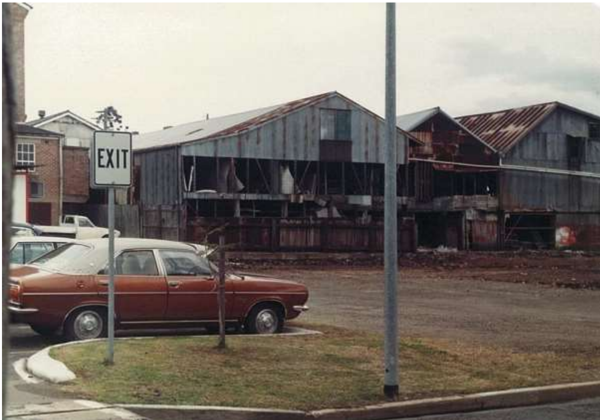
FIGURE 2.42 – PRYOR'S PLASTERWORKS IN 1983 PRIOR TO DEMOLITION LOOKING NORTH-EAST FROM GRANT STREET
