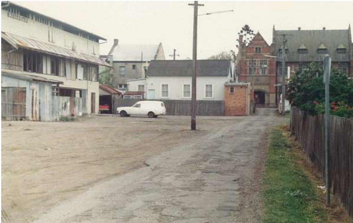
FIGURE 2.41 – PRYOR'S PLASTERWORKS 1983 PRIOR TO DEMOLITION, LOOKING NORTH TOWARDS HIGH STREET. THIS PHOTOGRAPH PROVIDES A VIEW OF THE REAR OF BUILDINGS ALONG HIGH STREET
