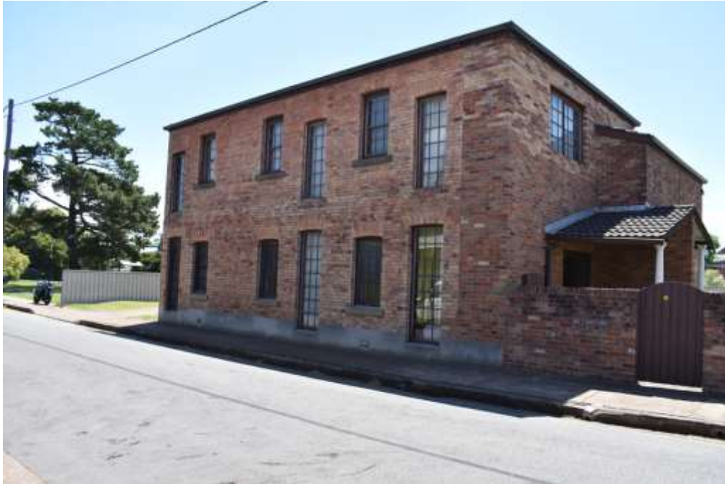
FIGURE 2.39 - TERRACES CONSTRUCTED CIRCA 1880S LOCATED ON LOT 5
