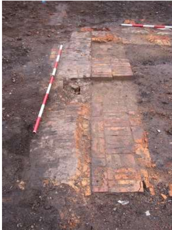
FIGURE 2.28 - REMNANT BRICKWORK LOCATED AT THE REAR OF 273 HIGH STREET THOUGHT TO BE ASSOCIATED WITH G J WEBBER, TINSMITH Source: Eureka, 2012.
