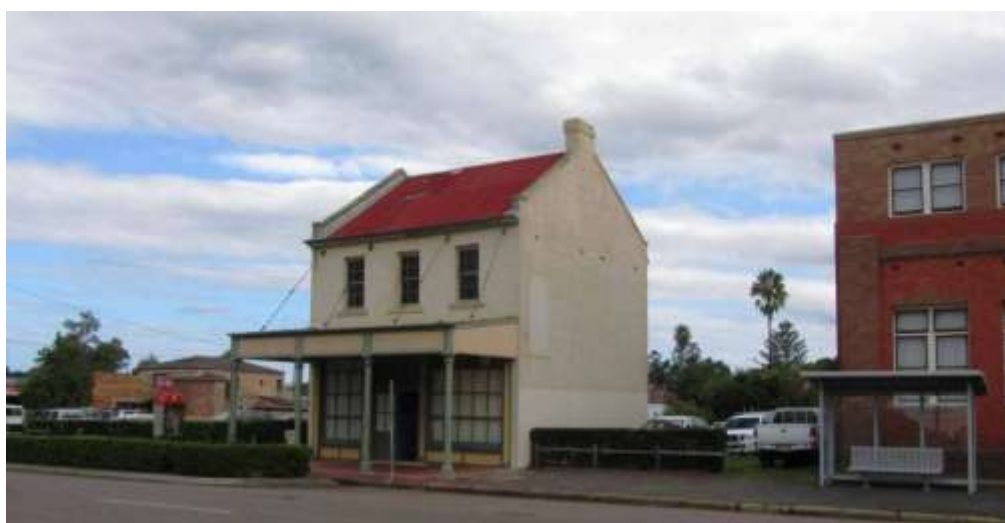
FIGURE 2.26 - LOOKING SOUTHERLY ACROSS HIGH STREET TO THE FORMER TOWN HALL CAFÉ BUILDING.
