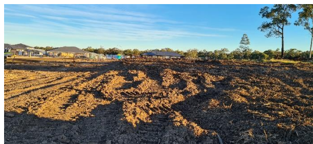
Photograph 8: Facing southwest from near TP504.
