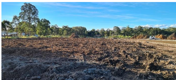
Photograph 5: Facing north from near TP501.
