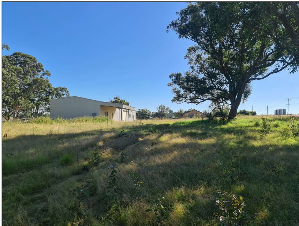
Photograph 2 – view of the site and storage shed from the south.
