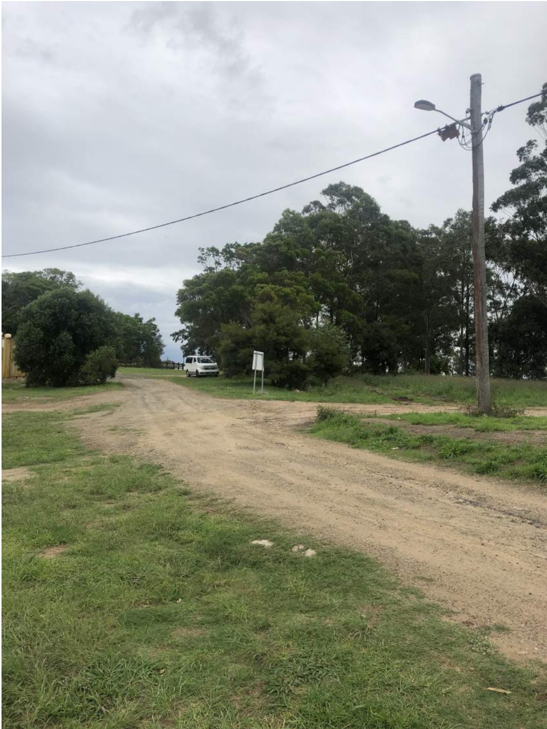
Figure 3: Photograph of the existing road; looking toward Morpeth House.
