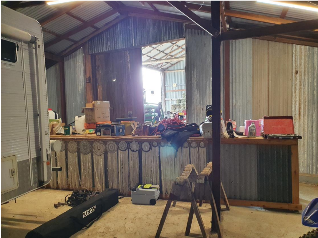
FIGURE 7: SHOWING LARGE DOOR TO CLASS 10A SHED
