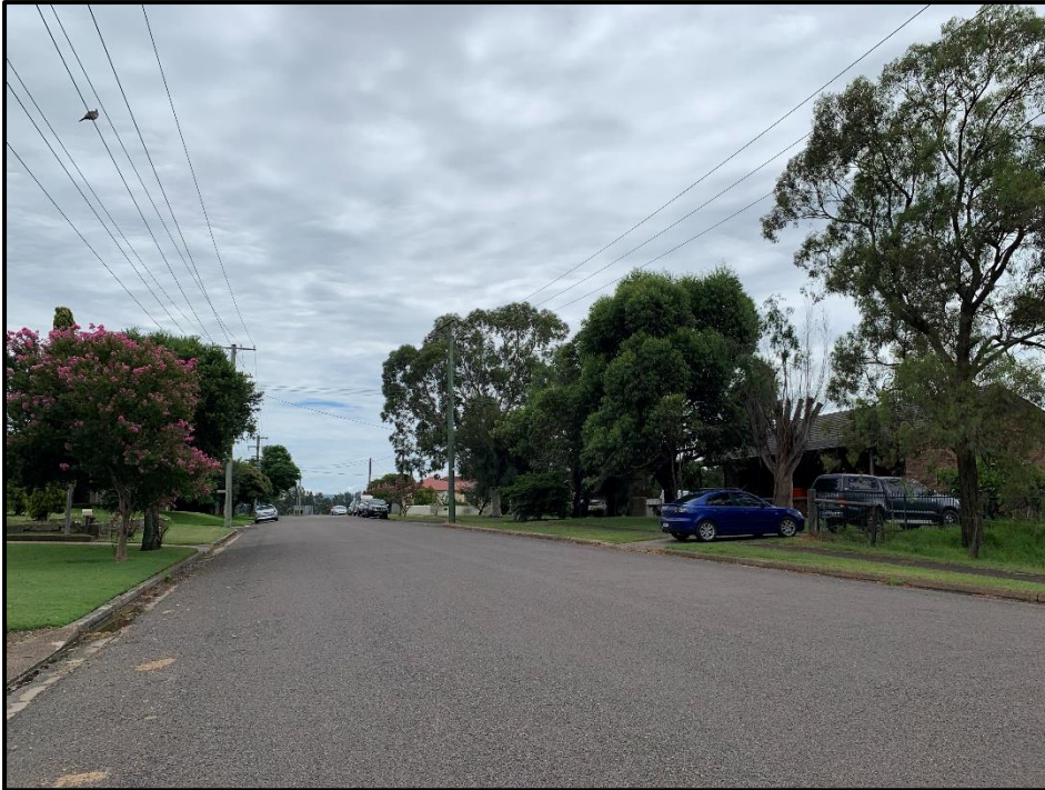
Photo 2 – View looking west along Edward Street showing typical cross section and alignment
