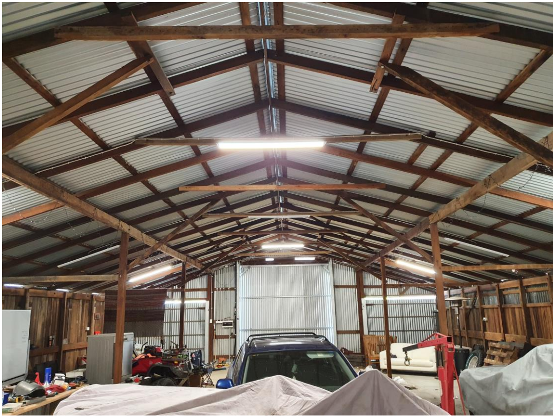
IMAGE 1: GENERAL FUNCTION CENTRE CONSTRUCTION
