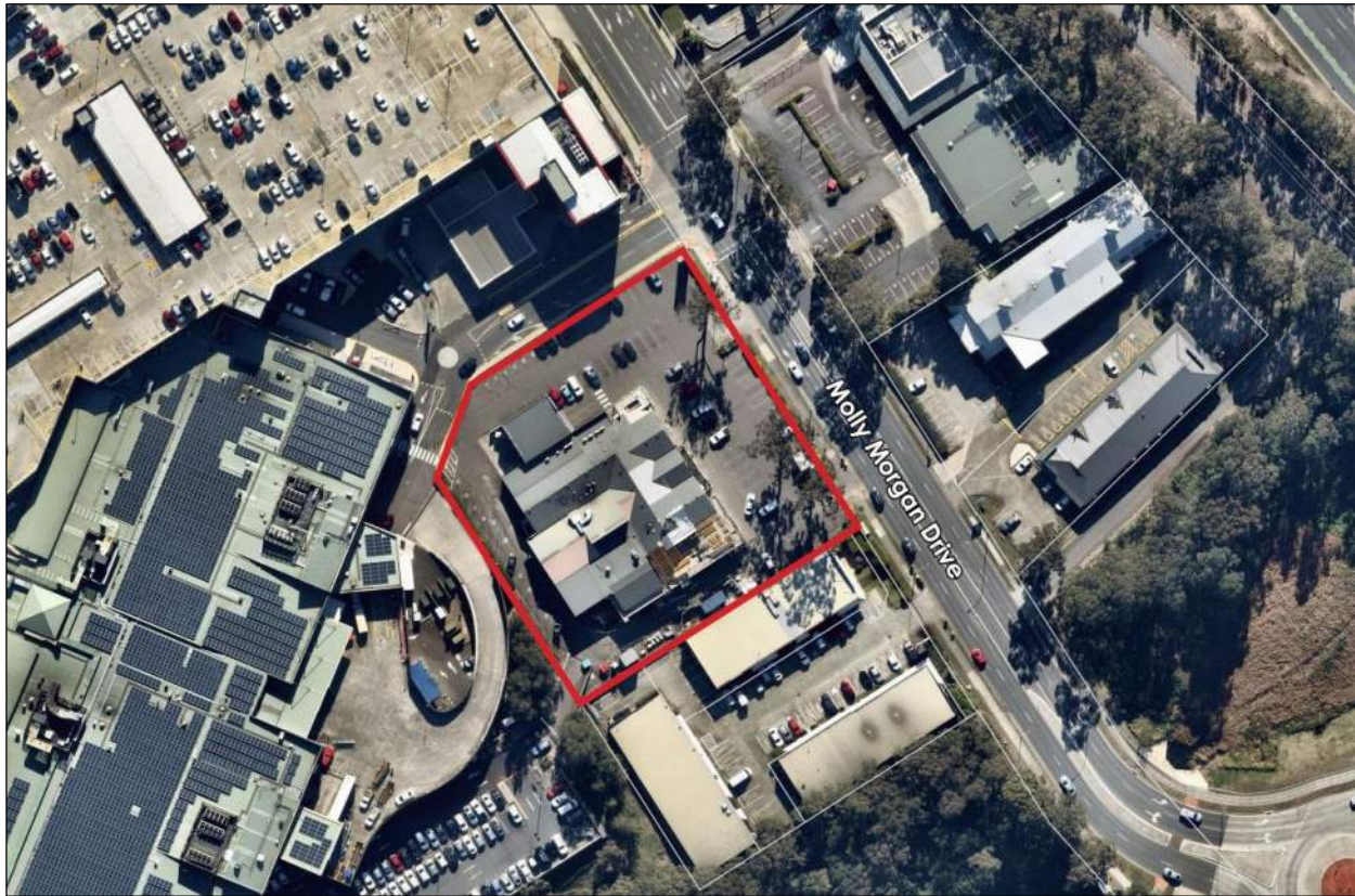
Figure 1 – Aerial photograph of Subject Site (outline red) (Source: Nearmap)
