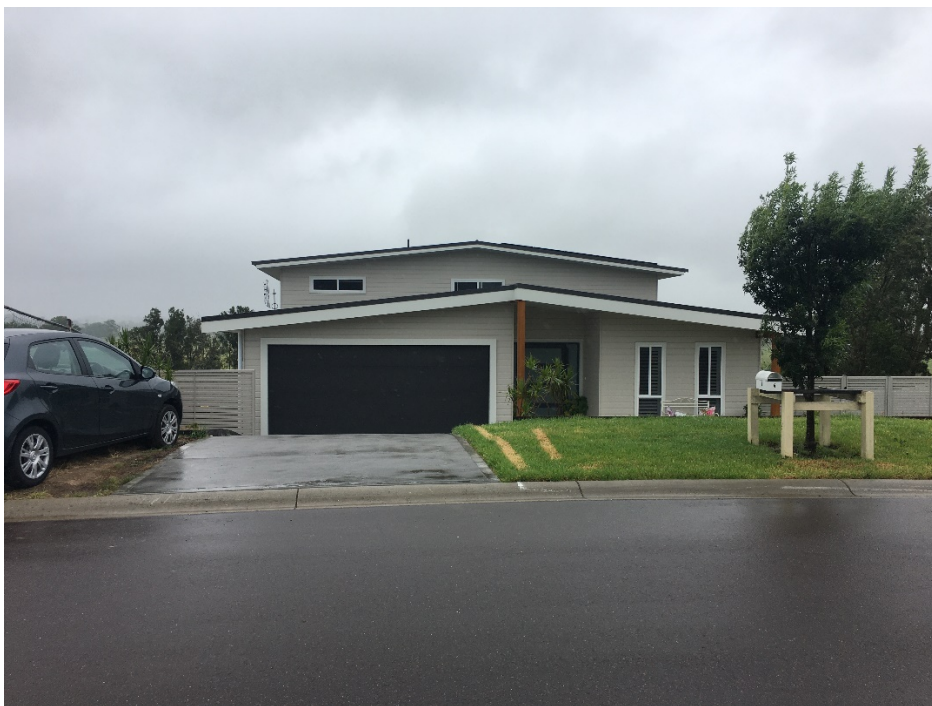
Figure 2: Two storey weatherboard dwelling, Riverside Street.
