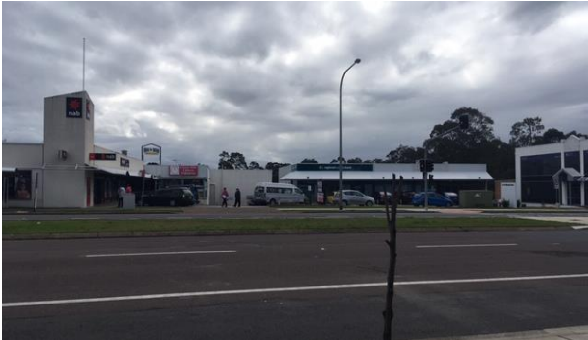
Figure 2 – Existing commercial buildings on site on Mitchell Drive East Maitland
