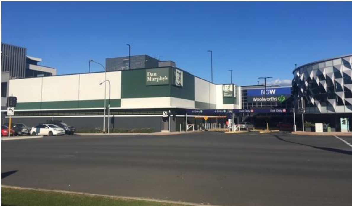
Figure 4 – Entrance to Stockland's Greenhills Shopping Centre opposite the site.
