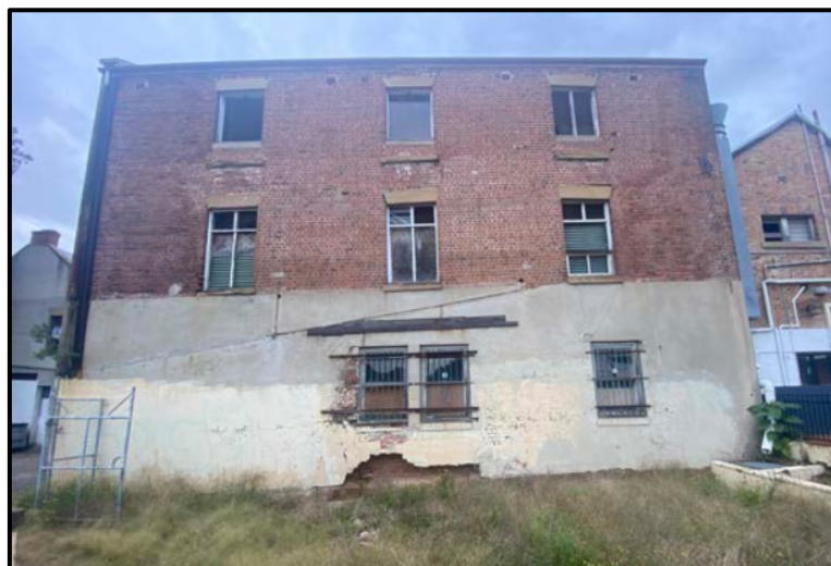
Figure 4: Northern elevation of existing building (Source: SOHI, caste Studio, 2022)
