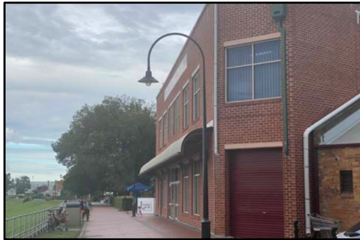
Figure 8: Eastern elevation of existing building (Source: SOHI, caste Studio, 2022)
