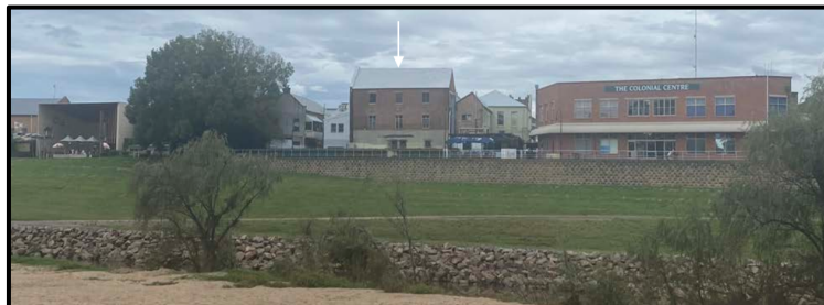
Figure 9: Eastern elevation of existing building (Source: SOHI, caste Studio, 2022)
