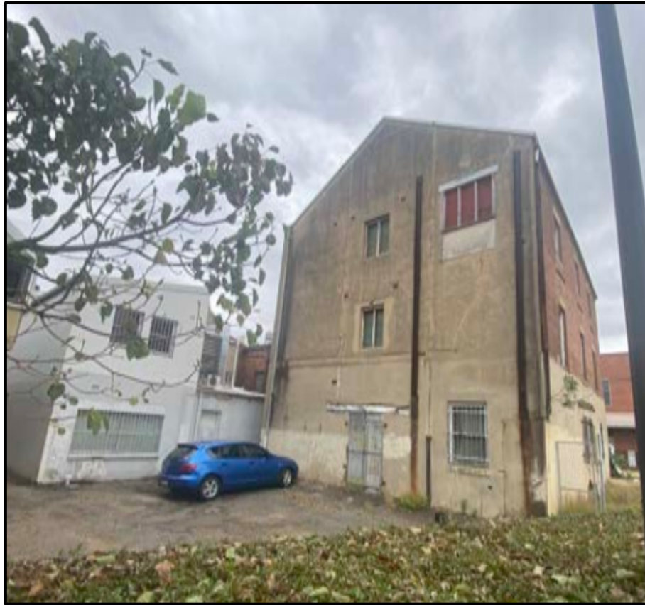
Figure 5: Eastern elevation of existing building (Source: SOHI, caste Studio, 2022)
