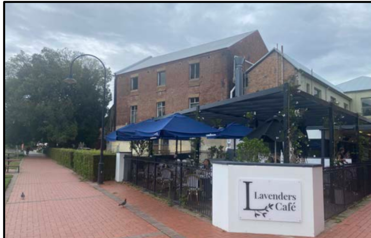
Figure 7: Eastern elevation of existing building (Source: SOHI, caste Studio, 2022)
