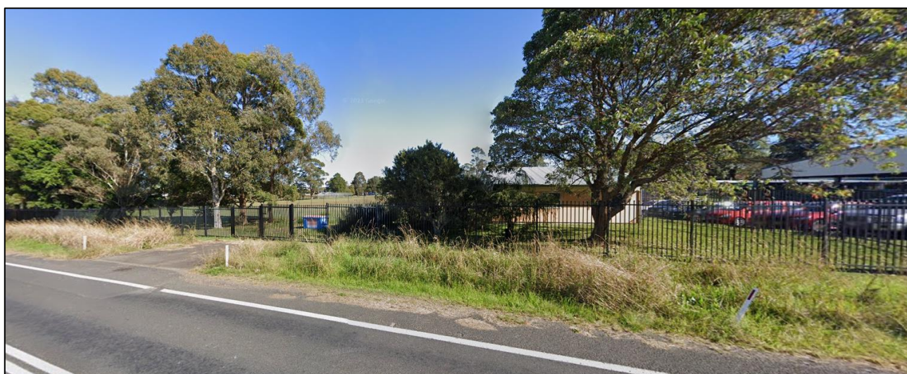
Photograph 5: View of area where car park is proposed from Woodberry Road (Source: Google Street View; May 2022)
