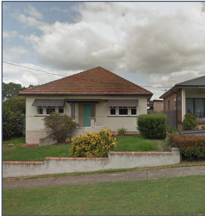
Figure 2: Existing dwelling at 277 Newcastle Street, East Maitland
