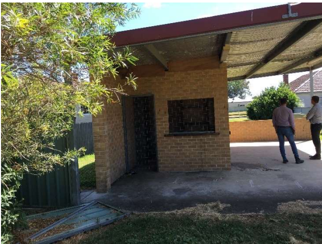
(Figure 5: Northern adjoining property fence)
