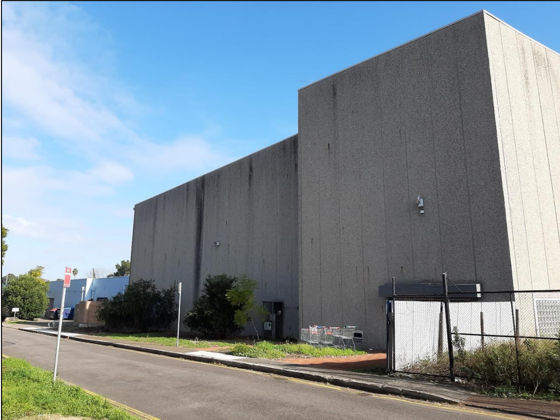
Figure 3 Adjoining Cinema Complex
