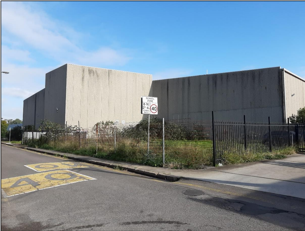
Figure 6 Subject Site as viewed from Lee Street
