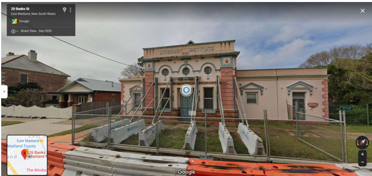
Figure 3: No.20 Banks Street a prominent and interesting heritage building. Very prominent parapet design elements and colour detailing, varied fenestration breakup and design.
