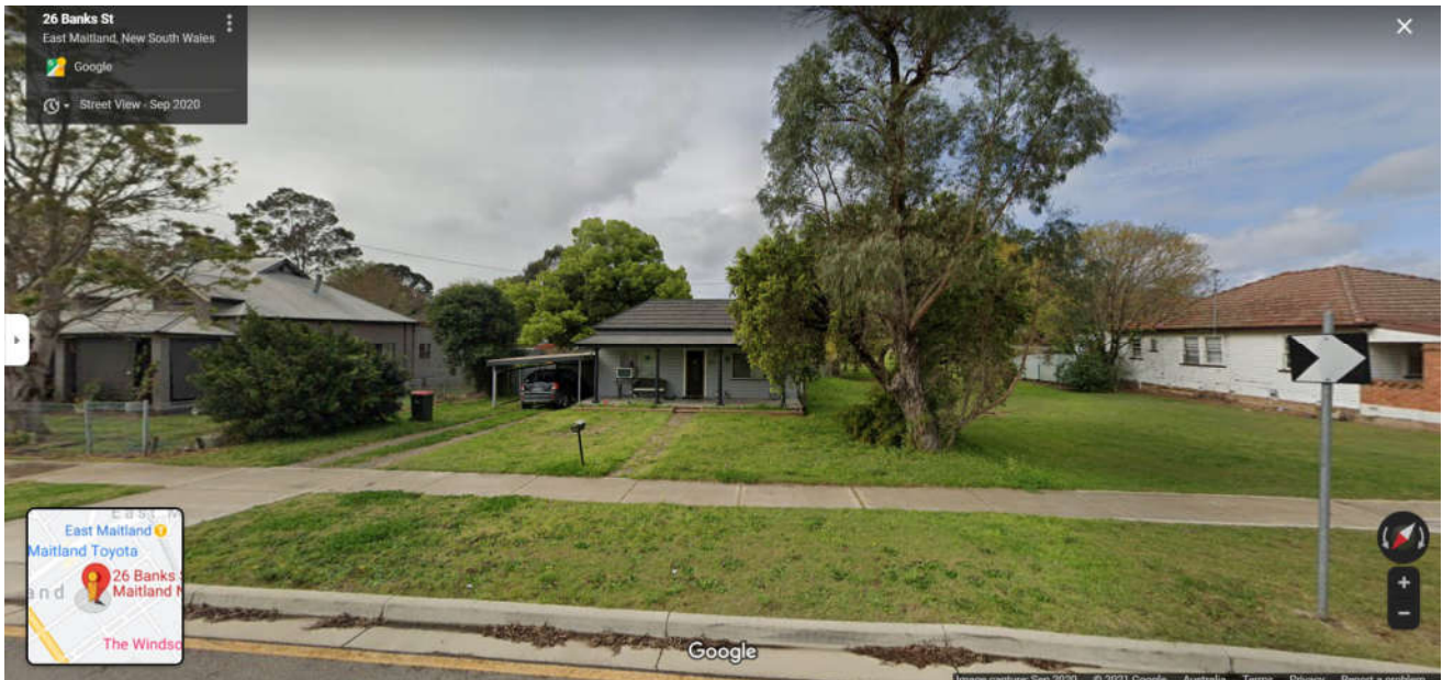
Figure 5: This picture shows existing 26 Banks Street Development site. Simple single level workers cottage.
