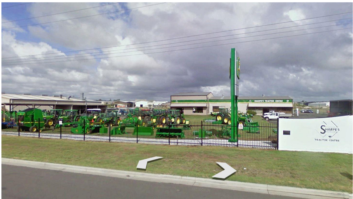
PHOTO 1 – View of Facility from Racecourse Road
