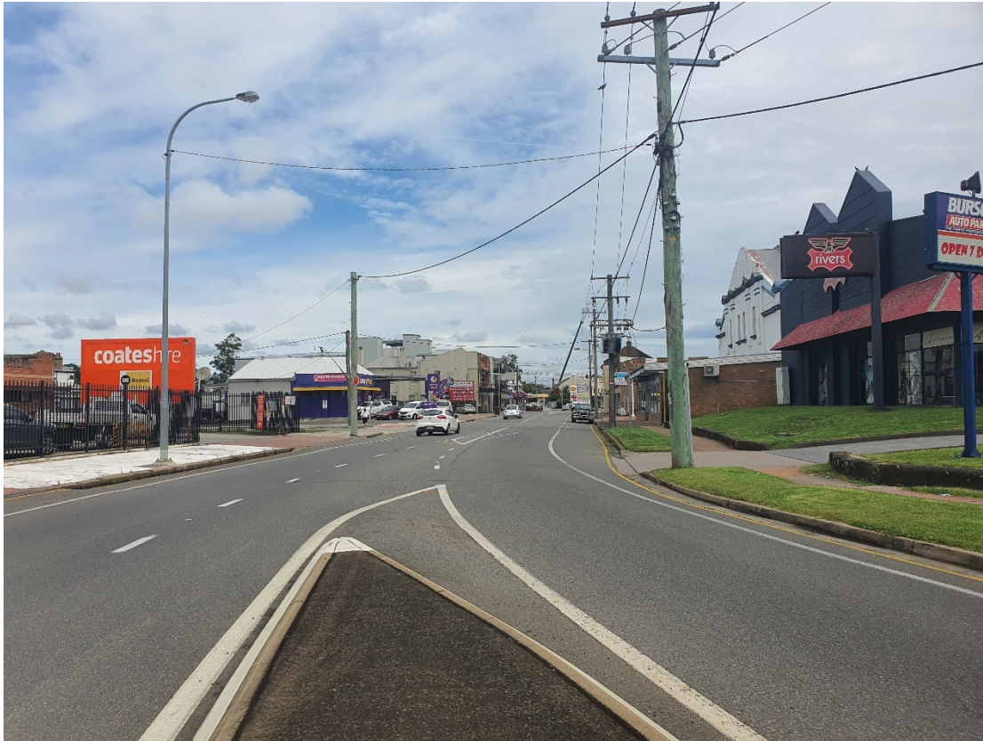
Image 40 Central Median before railway overpass
