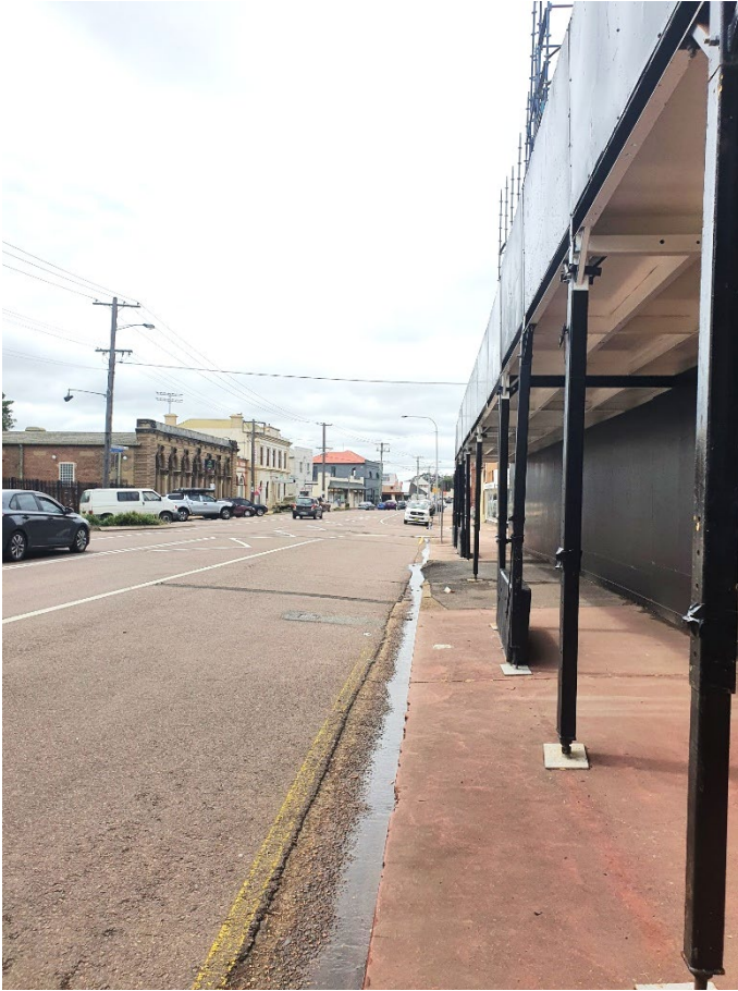
Image 29 New Maitland Administration Centre Site
