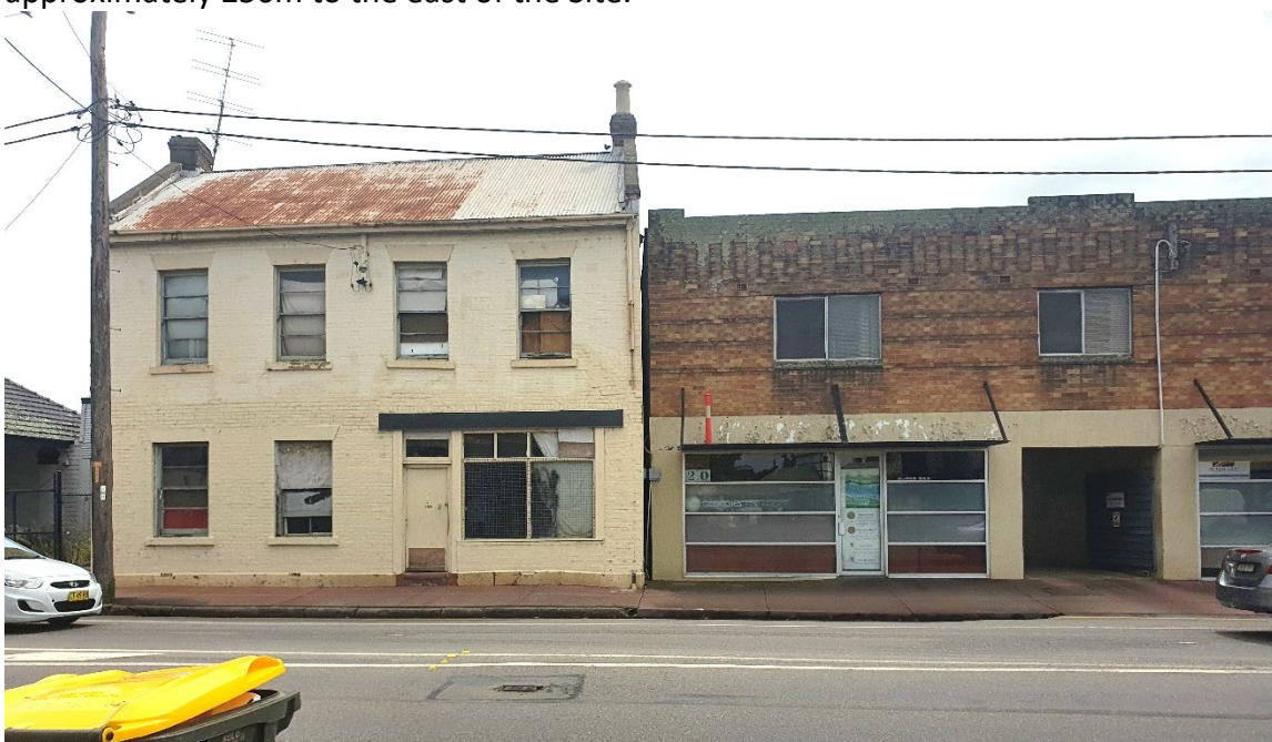
Image 41 Eastern boundary of the Site
