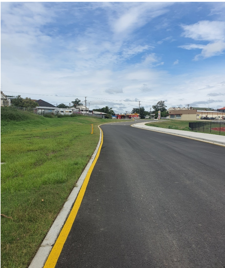
Image 51 Looking south west along the Sportsground access
