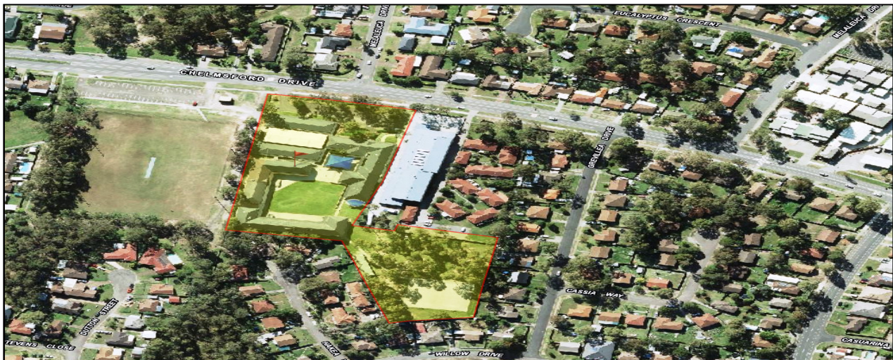
FIGURE 6- EXISTING SCHOOL IMPROVEMENTS- AERIAL IMAGE
